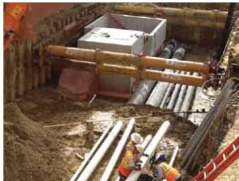
Groundforce hydraulic struts support sheet pile shoring system, providing safety to project teams.
