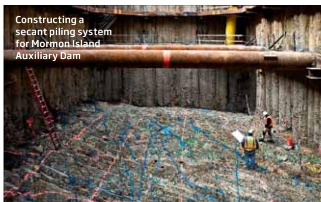
Constructing a secant piling system for Mormon Island Auxiliary Dam
