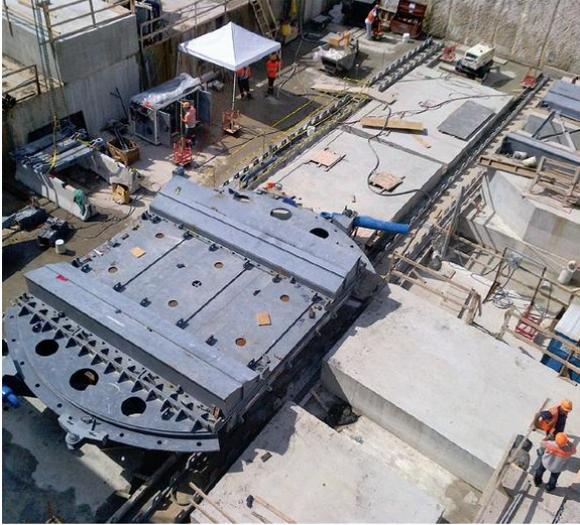
Crews slid Harriet's "head" off the body of trailing gear and onto a Teflon turntable that slowly rotated it around to face the opposite direction. Then, the trailing gear was re-attached, and tunneling began again.
