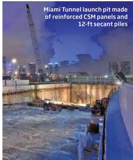
Miami Tunnel launch pit made of reinforced CSM panels and 12-ft secant piles
