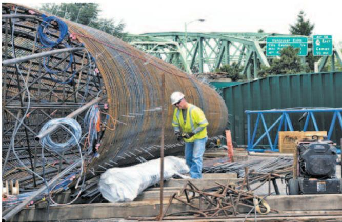
Cage with testing apparatus.
