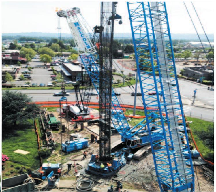
to arrive at a timely solution. A decision was made that required the shaft to be backfilled with gravel, and the casing removed. The tooth ring was repaired, reinforced, and installation of the shaft
