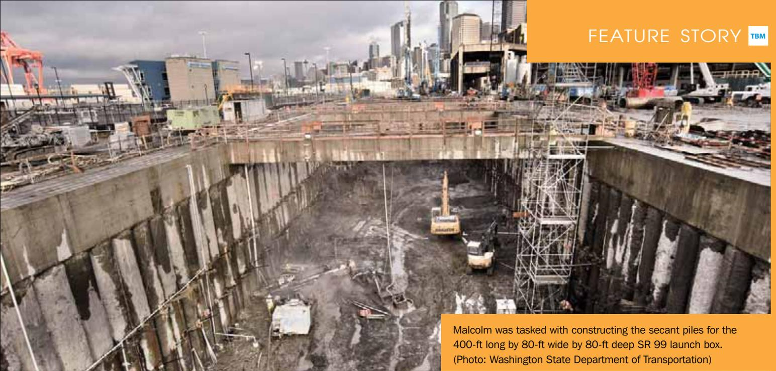
Malcolm was tasked with constructing the secant piles for the 400-ft long by 80-ft wide by 80-ft deep SR 99 launch box. (Photo: Washington State Department of Transportation)
