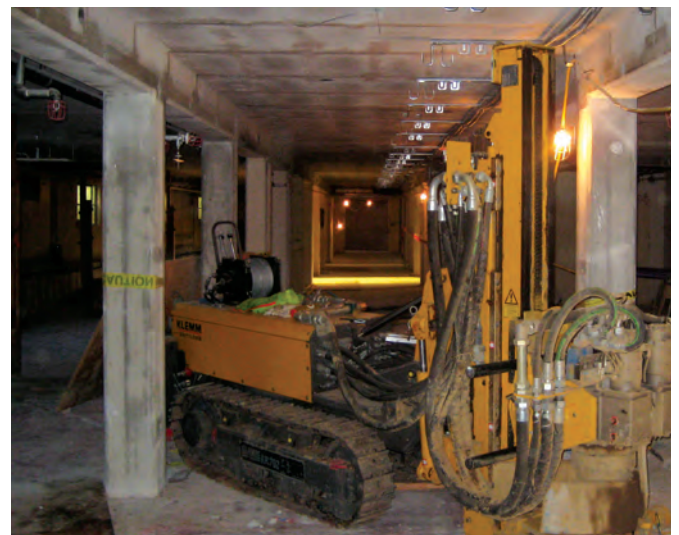
OPPOSITE: Restricted Access Drill Rig LEFT: Tiedowns, San Francisco, CA BELOW: Low Headroom Drilling
