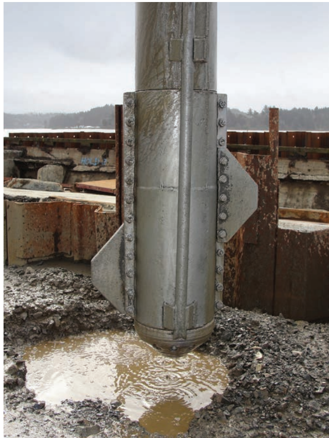
BELOW: Vibrocompaction, Port of Newport, OR
