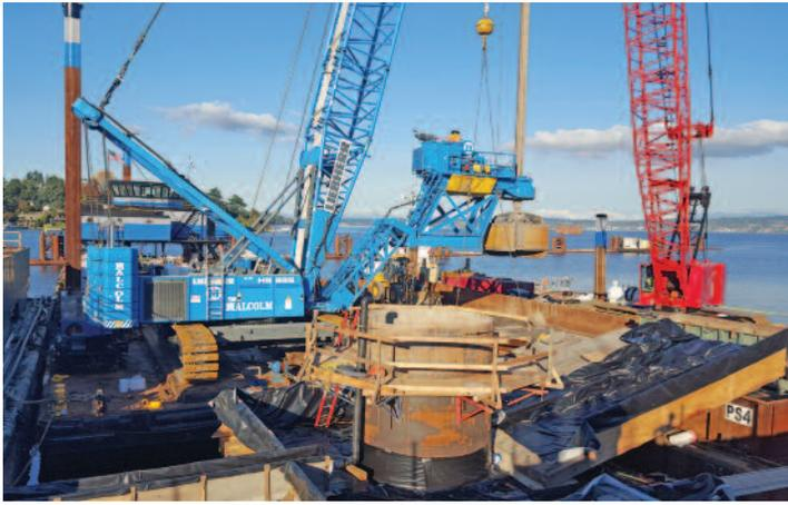
Drilling slurry was also utilized on this project and needed to be piped using high density polyethylene (HDPE) piping and was wrapped with secondary containment in high traffic areas. A group of plumbed baker tanks followed the operations down the trestle allowing for storage, batching and remixing.
