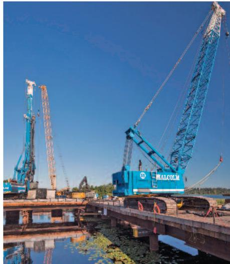
Questions evolved from how to drill the shafts to how we would be able to access the shafts and ensure that the environment below wasn't impacted by the construction operations. Steel pipe piles and 12"x12" timber with finger sections that projected off towards each shaft were used to support cranes, drill rigs and provide access for spoils hauling and concrete and extended over 2,000 lin-
