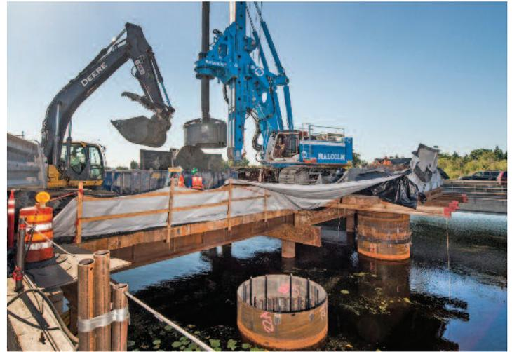
feet. The trestle that was constructed covered the structural needs to access the work areas but didn't account for containment.
