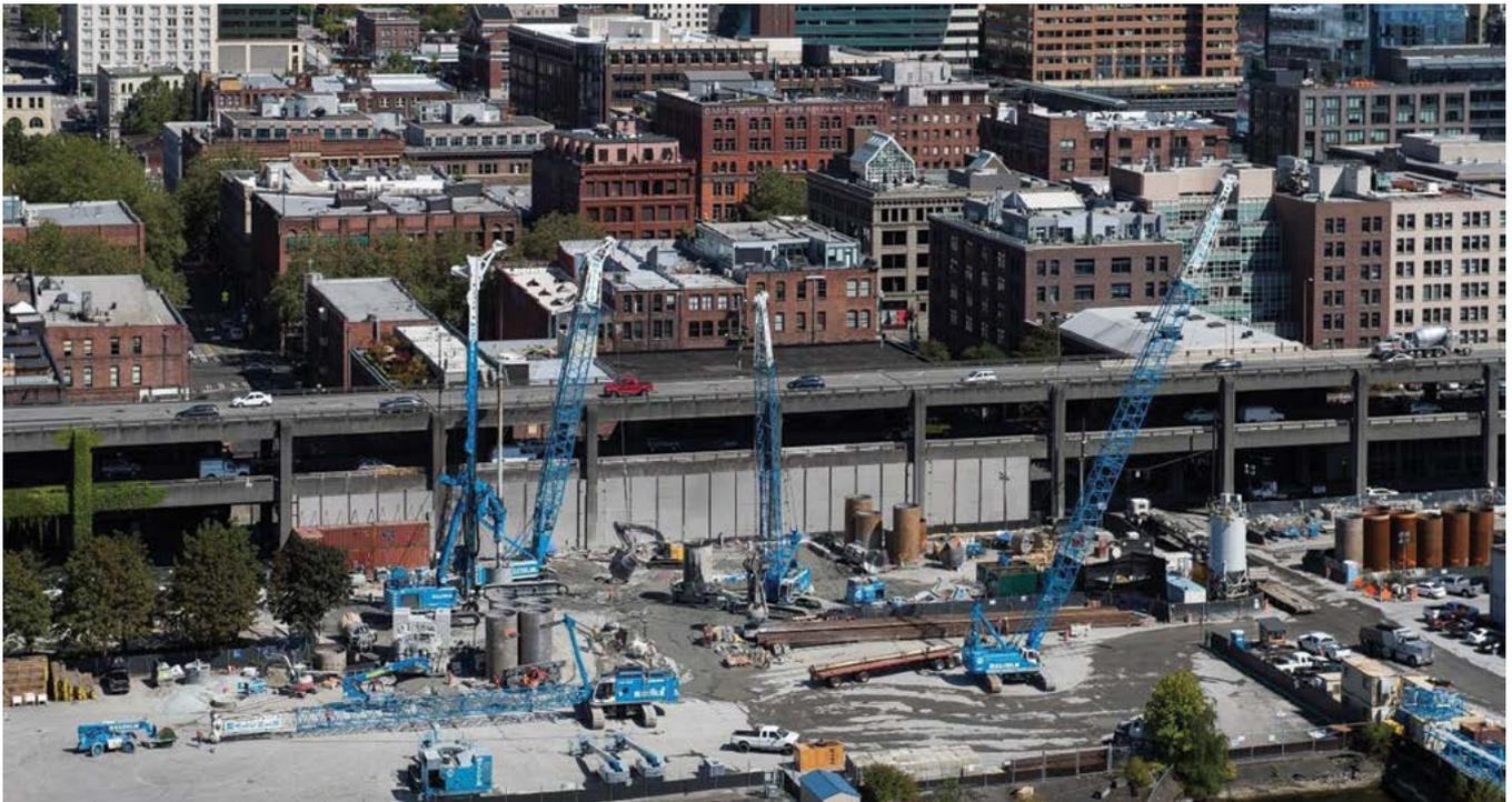
**M**ining on Seattle's SR99 tunnel began in July of 2013. Initial mining progressed slowly through a 4.5 m (14.9-ft) thick fiber-reinforced concrete headwall before immediately entering the first of three planned safe havens. Once through the headwall and safe haven the machine would move through roughly 122 lineal m (400 ft) of jet grout improved soil at a rate of slightly more than 1.6 m/d (5.3 ftpd). It was anticipated
