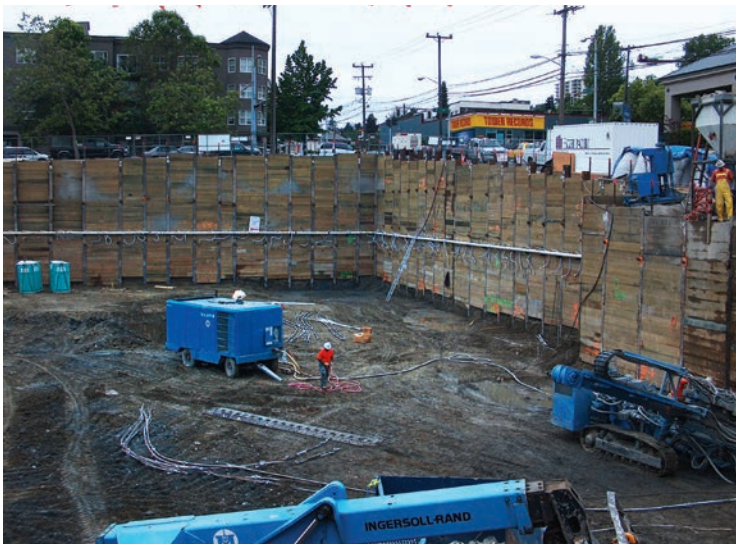
TOP LEFT: Vacuum wellpoints installed through the shoring wall in order to reach excavation depth and still lift the water out of a deeper excavation. BOTTOM LEFT: Vacuum wellpoint system hung on shoring wall. RIGHT: Vacuum wellpoints closely spaced due to nearby river.
