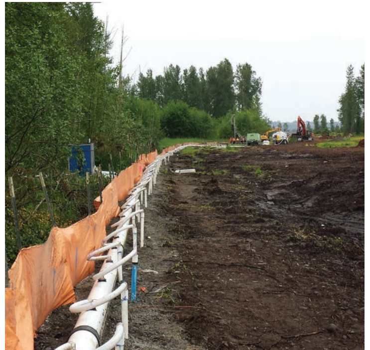
TOP LEFT: Vacuum wellpoints installed through the shoring wall in order to reach excavation depth and still lift the water out of a deeper excavation. BOTTOM LEFT: Vacuum wellpoint system hung on shoring wall. RIGHT: Vacuum wellpoints closely spaced due to nearby river.
