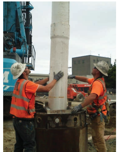
BOTTOM RIGHT: Installing 12-inch PVC well screen into a fully cased well.
