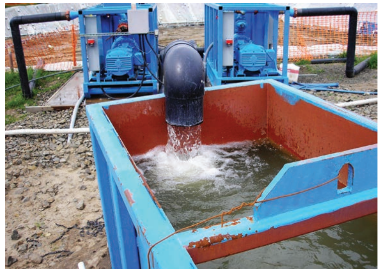
OPPOSITE: Eductor well system installed around a proposed future excavation. TOP LEFT: Eductor system manifold and pump. BOTTOM LEFT: Eductor system manifold wrapped around 30-foot-deep excavation. BOTTOM RIGHT: Eductor pumps and settlement tank.
