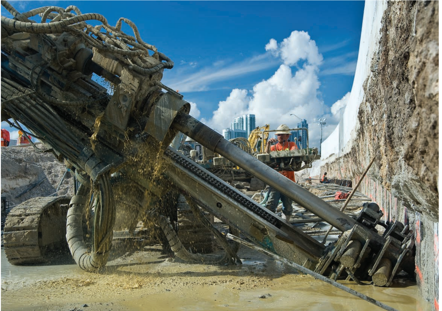
FRONT COVER: Internal bracing, Oceanwide Center, San Francisco, CA BACK COVER: Tieback anchor drilling, Miami, FL
