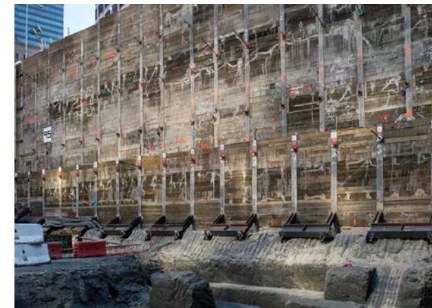
OPPOSITE: Tieback testing, anchored pile and timber lagging wall, Palo Alto, CA TOP LEFT: Anchored pile and timber lagging wall, Los Angeles, CA BOTTOM LEFT: Internally braced pile and timber lagging, Palo Alto, CA RIGHT: Anchored pile and timber lagging wall, San Francisco, CA
