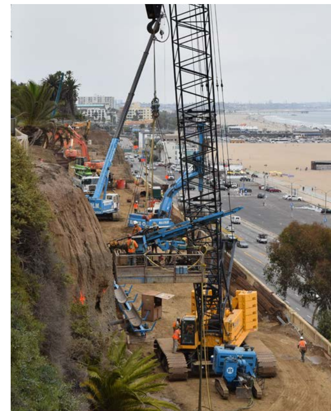
OPPOSITE: Anchored stitched piers, Big Sky, MT LEFT: Suspended drilling platform, Santa Monica, CA RIGHT: Slope anchorage, Orange County, CA
