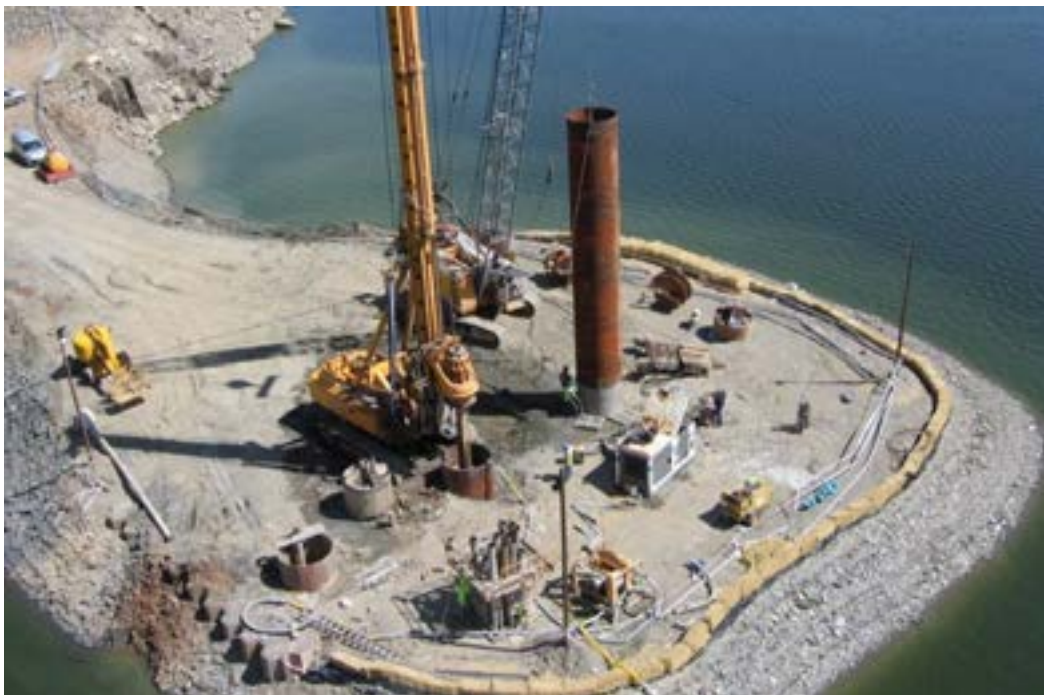
Fig A8. Example of edge protection around the platform to protect the environment
