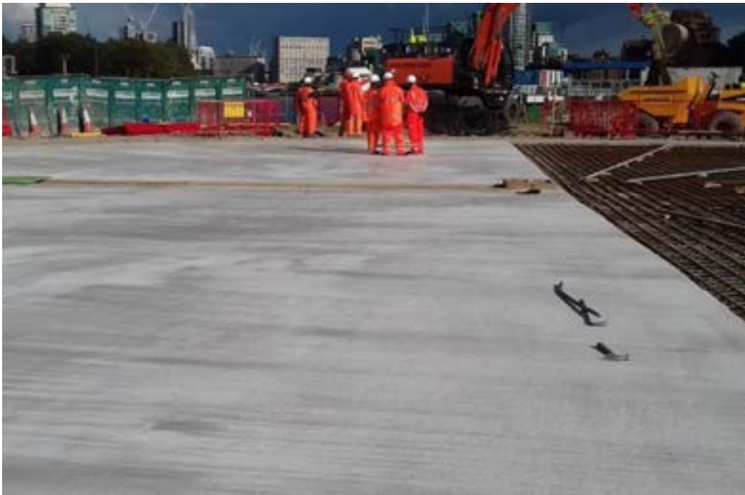
Fig A7. Example of a reinforced concrete platform (with drainage in centre)
