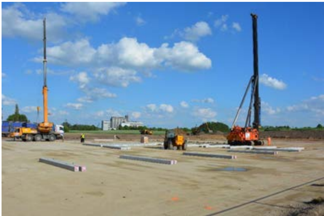
Fig A6. Example of a cement bound platform (level smooth surface – beware of ponding)
