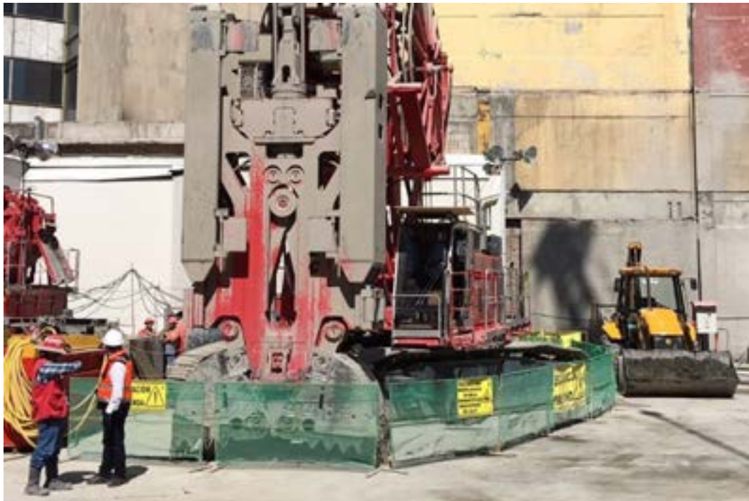
Fig A3. Example of a concreted platform
