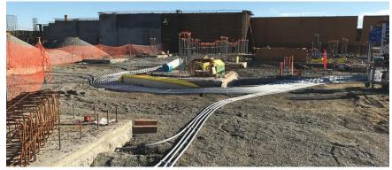
The largest geothermal pile system in the U.S. has nearly 100 miles of pipes and the equivalent of 12 American football fields of covered surface area.
