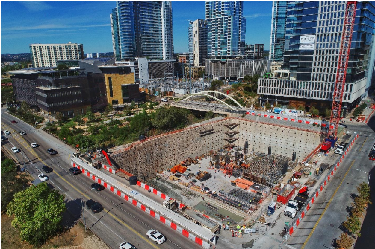
Figure 17. Aerial view of the completed diaphragm wall and excavation.
