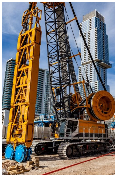
Figure 12. BC40 Hydromill mounted on MC96 crane.
