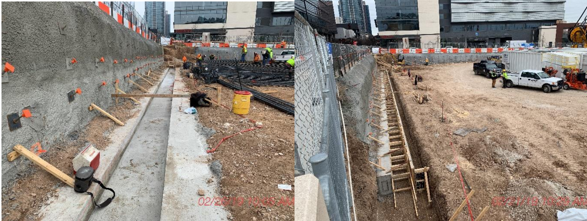
Figure 11. Guide wall construction.
