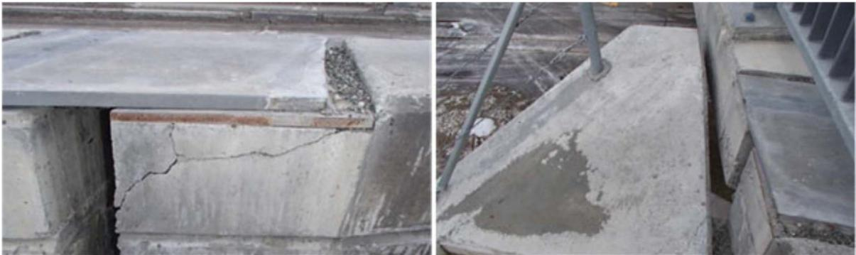
**Fig. 39. Photographs at the northeast transition from the bridge span to the approach fill showing evidence of possible pounding and permanent transverse displacements (courtesy of D. Hemstreet, from GEER 2018)**
