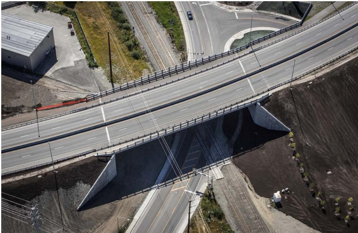
**Fig. 28. West Dowling Road Overcrossing near completion (Photo courtesy of HDR; ©2020); note the spur road crossing under the south approach fill (upper right corner of photograph)**
