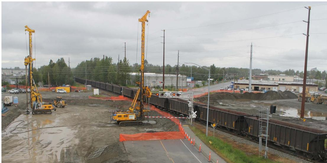
**Fig. 32. Deep mixing at the west approach abutment; minimum clearance of 6 m between DM columns and the active Alaska Railroad (Yamasaki et al. 2015)**
