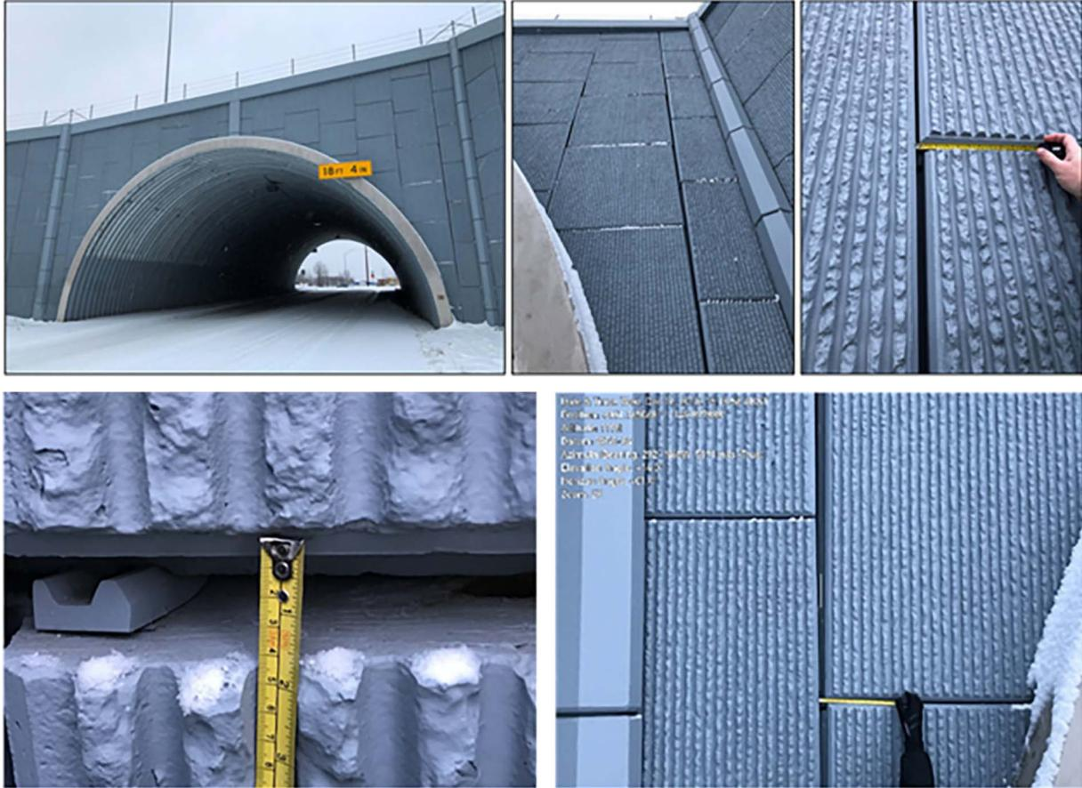
**Fig. 40. MSE walls around the culvert tunnel immediately south of the West Dowling Road Overcrossing: close ups illustrate panel movements, panel tilts, and unloading of a bearing pad (GEER 2018)**
