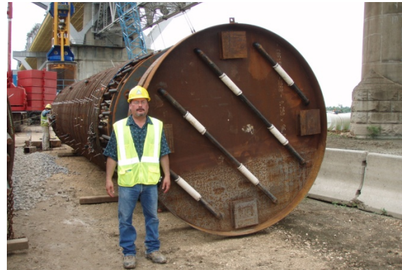
Figure 9: Sleeve-port Base Grouting System
