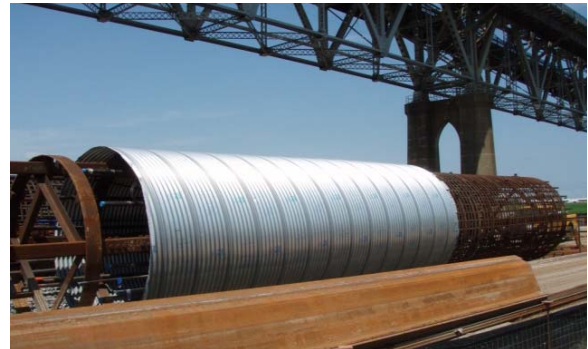
Figure 12: Isolation Casing Attached to Uppermost Section of Reinforcing Cage
