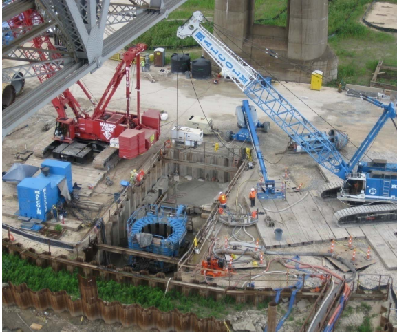
Figure 5: Rotator Placed into Excavation within the Working Platform
