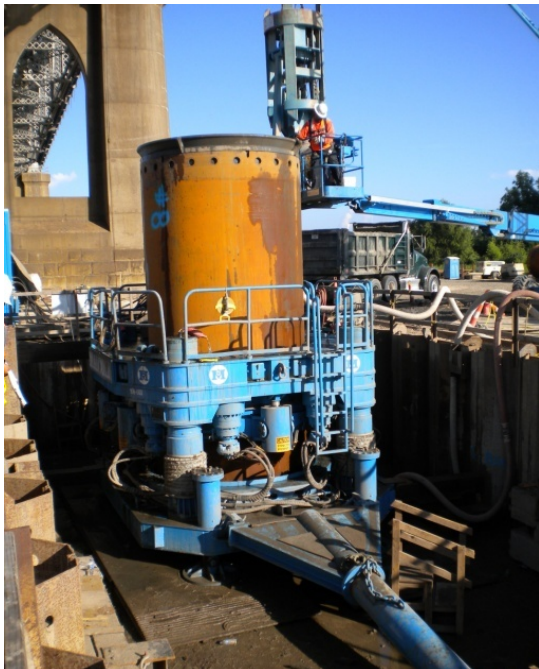
Figure 6: Rotator with Segmental Casing, using Excavation Support as Reaction
