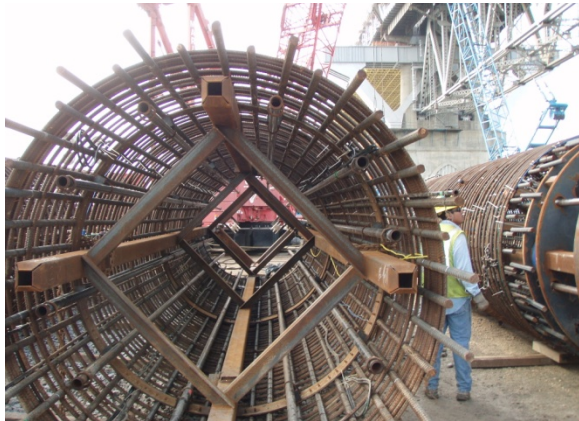
Figure 10: Back-bone Frame for Reinforcing Cage
