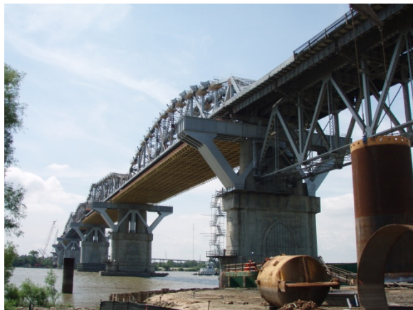
Figure 1: Huey P. Long Mississippi River Bridge (Pier IVA on Right).
