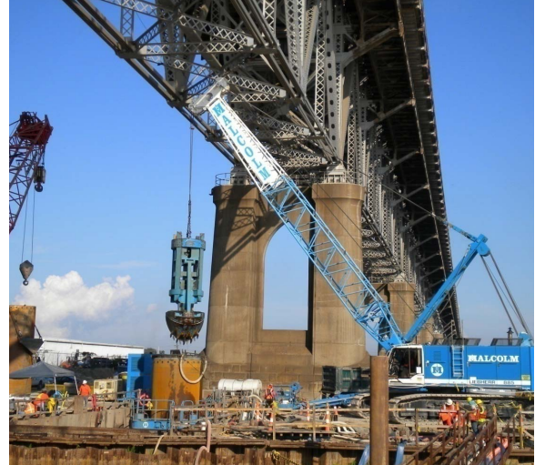
Figure 7: Excavation within the Casing Using a Hammer-grab
