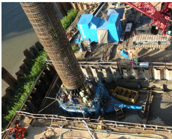
Figure 11: Splicing Reinforcing Cage
