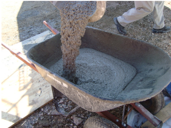
Figure 13: Drilled Shaft Concrete with Good Workability
