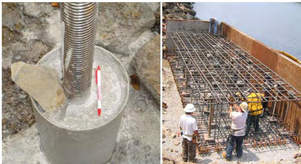
Figure 4 Completed Micropile and Connection to Footing
