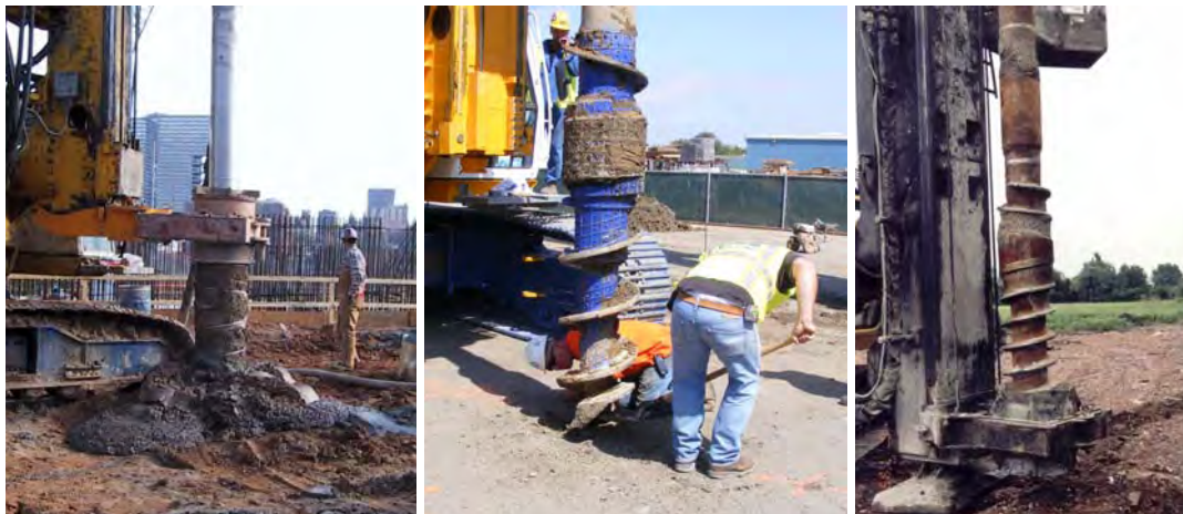
Figure 9 Drilled Displacement Tools
