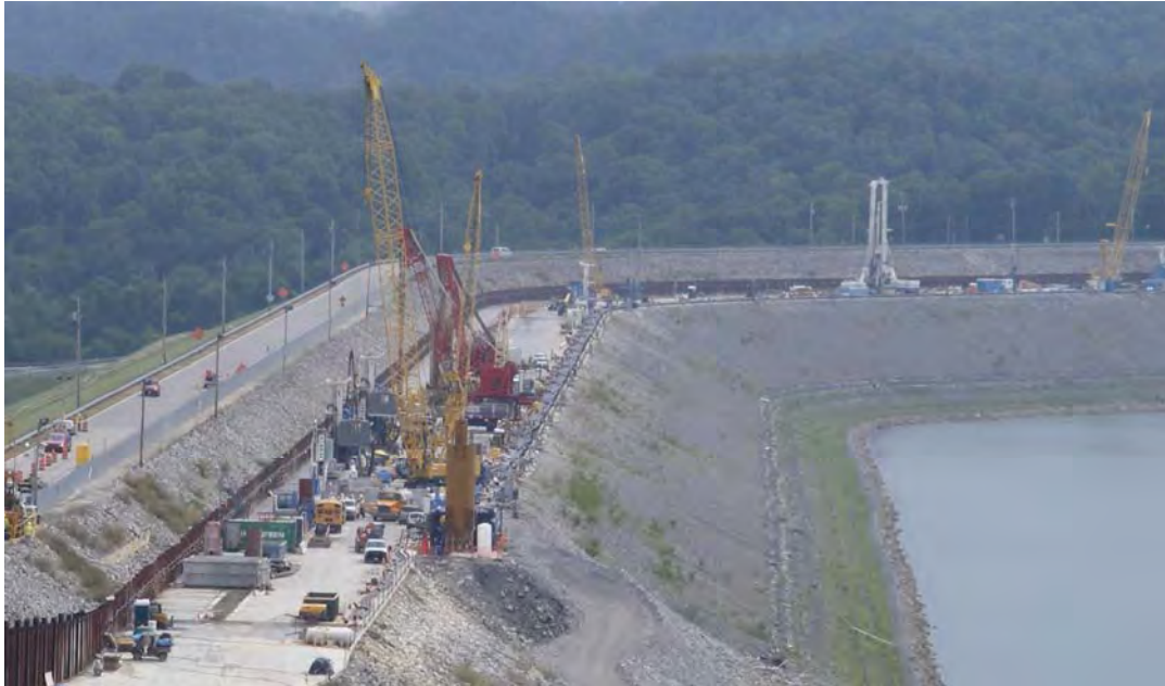
Figure 15 Work Platform at Wolf Creek Dam
