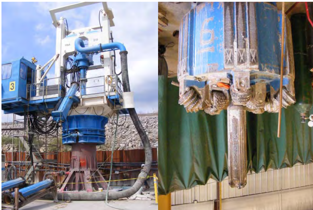
Figure 15 Reverse Circulation Drilling for Secant Pile Cutoff Wall
