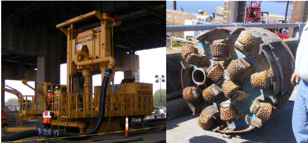
a) Restricted Headroom Drilling
