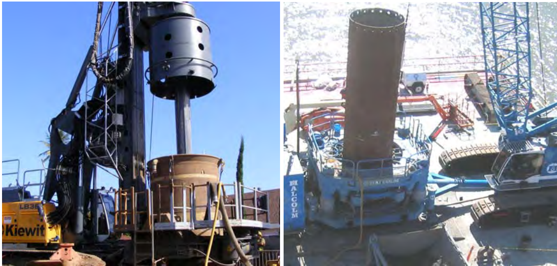
a) Drill-Mounted Oscillator
