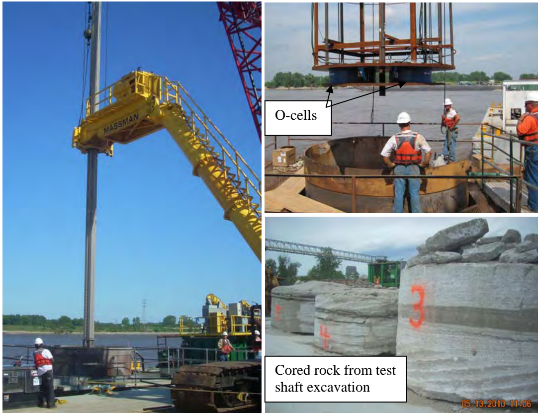
Figure 20 Load Test Shaft for the Mississippi River Bridge, St. Louis
