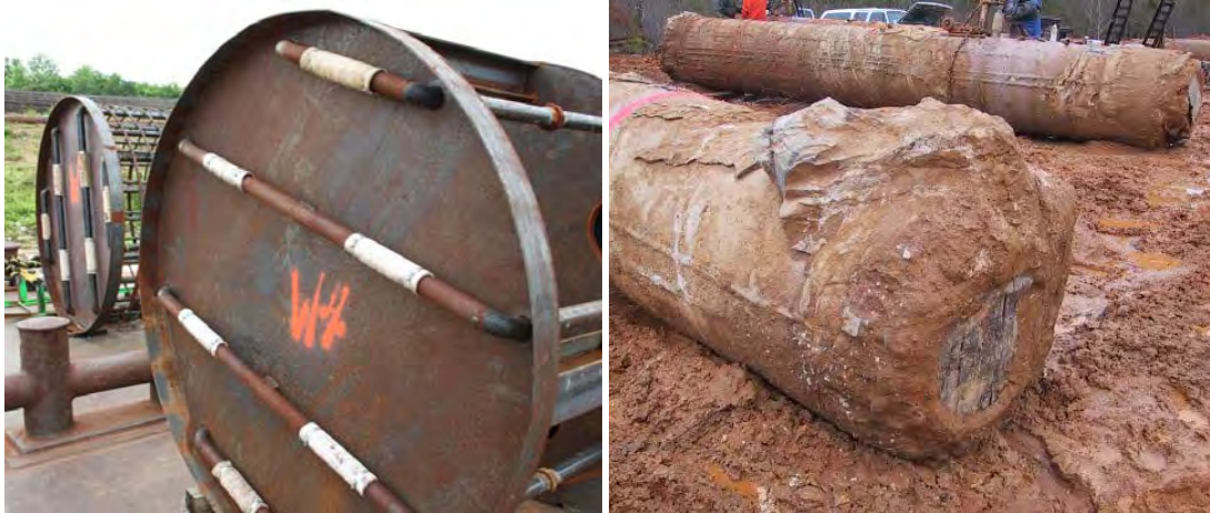
a) Sleeve Port System for Grouting
