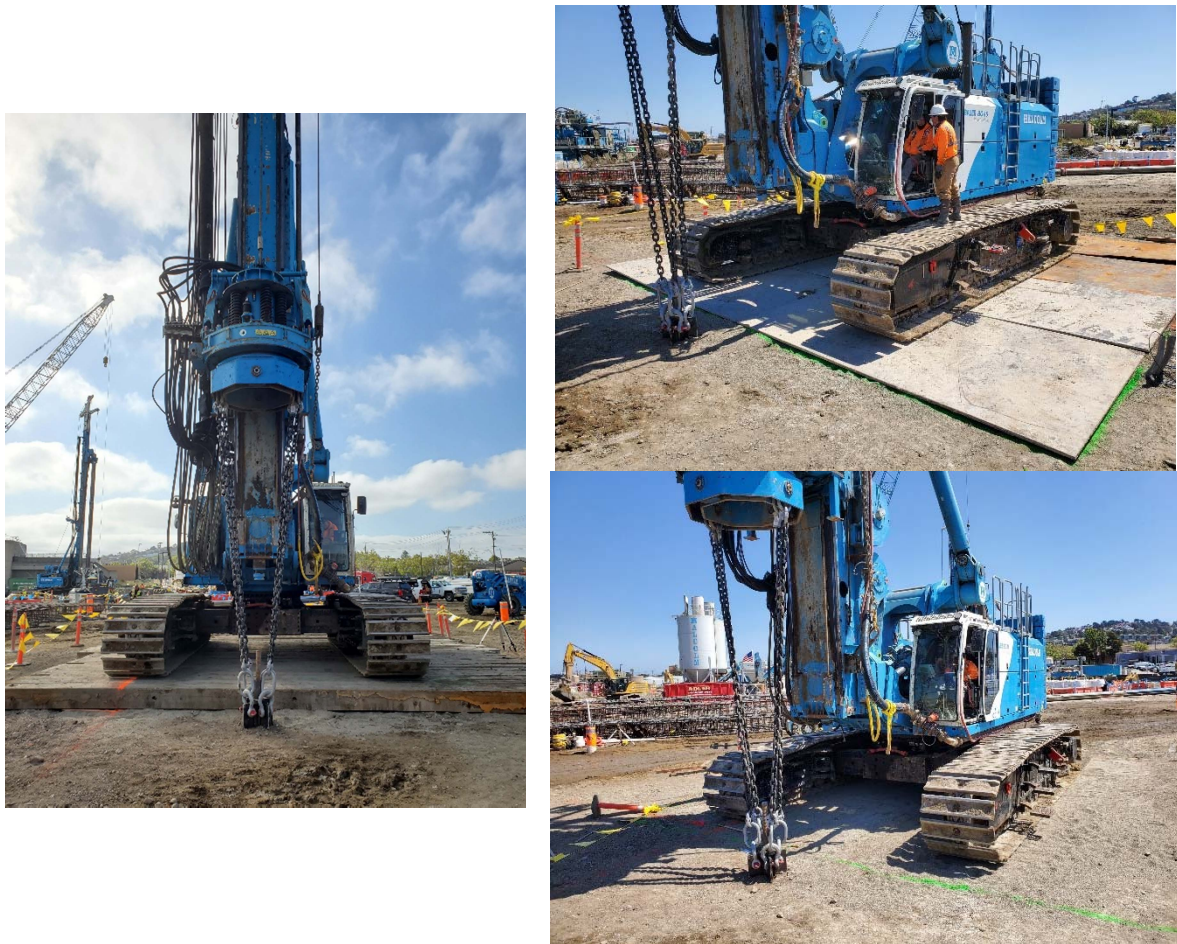
Figure 1. BG46 drilling machine with 3 different testing configurations
