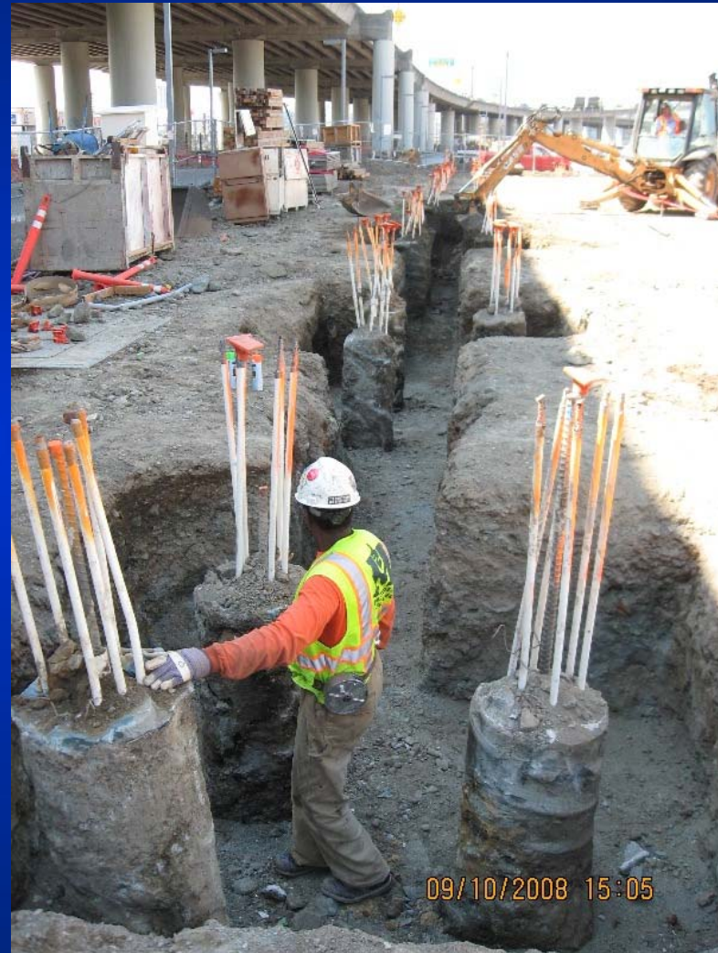
Pile Cap Work
