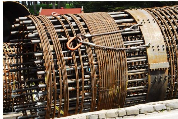
Figure 11: Rebar Stiffener Rings
