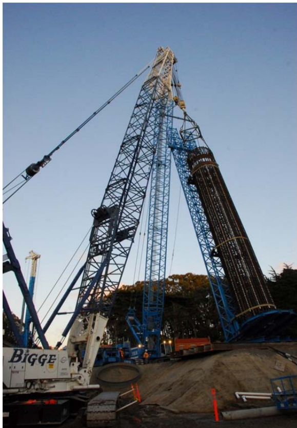
Figure 10: Rebar Cage Tipping Frame
