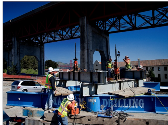
Figure 12: Rebar Suspension Frame
