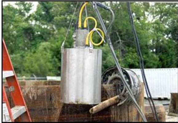
Figure 16: Shaft inspection Device (SID)
