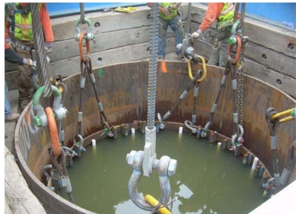
Figure 13: Rebar Cage Suspension
