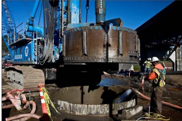
Figure 9: Rock Drilling Operation
