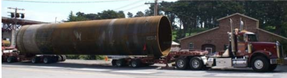
Figure 6: 12 foot Diameter Permanent Casing Section
