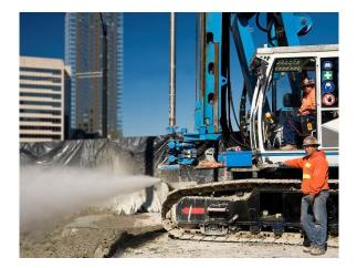
Figure 2: BG 15 with jet grouting attachment
