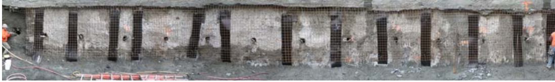
FIG. 7. Condition of Jet Grout Face for Lift 5.
