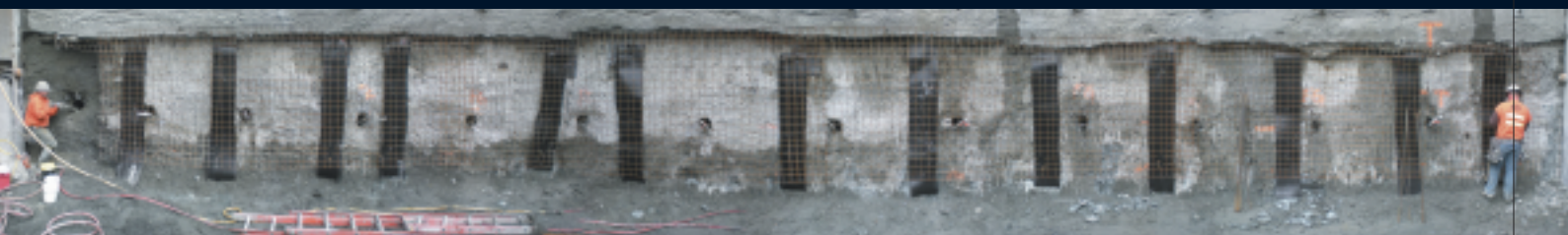
Figure 6: Condition of Jet Grout Face for Lift 5
