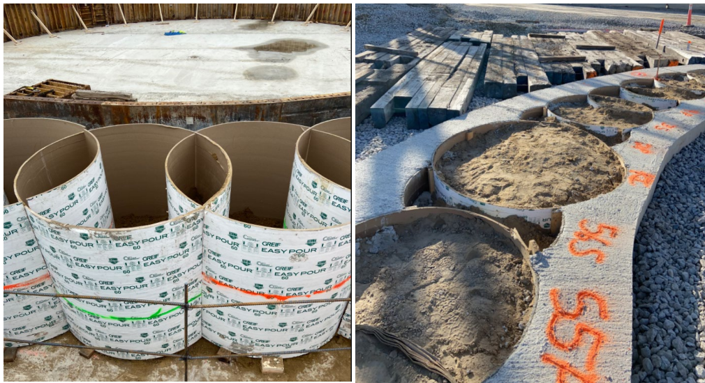
Figure 6 - Guidewall Construction Details
