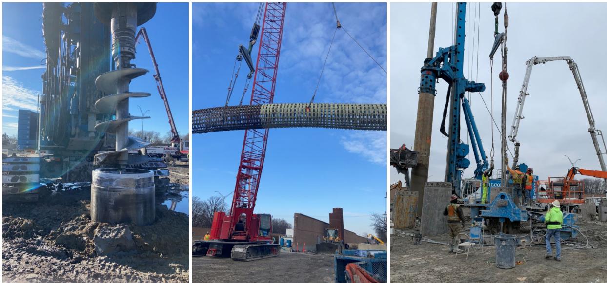
Figure 9 - Excavation, Composite Cage Placement, and Concreting
