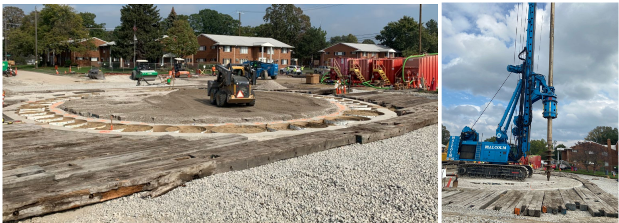
Figure 5 - Working Platform Construction
