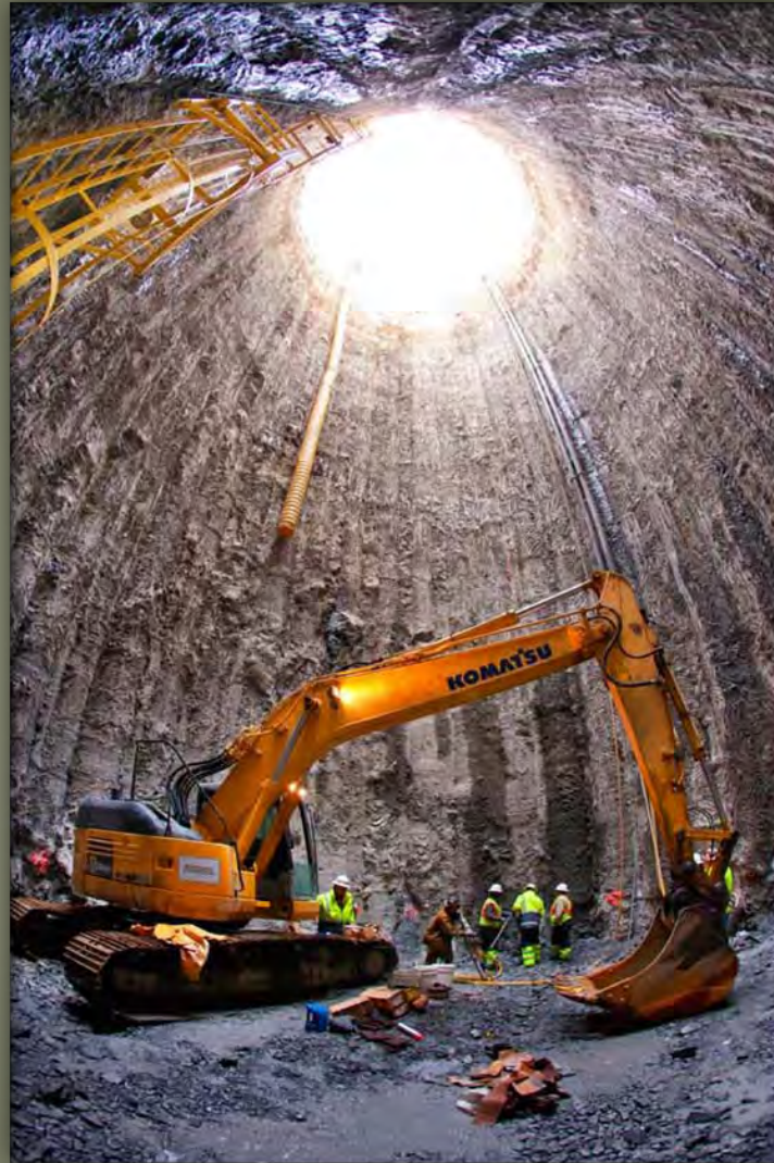
Shaft at Full Depth
