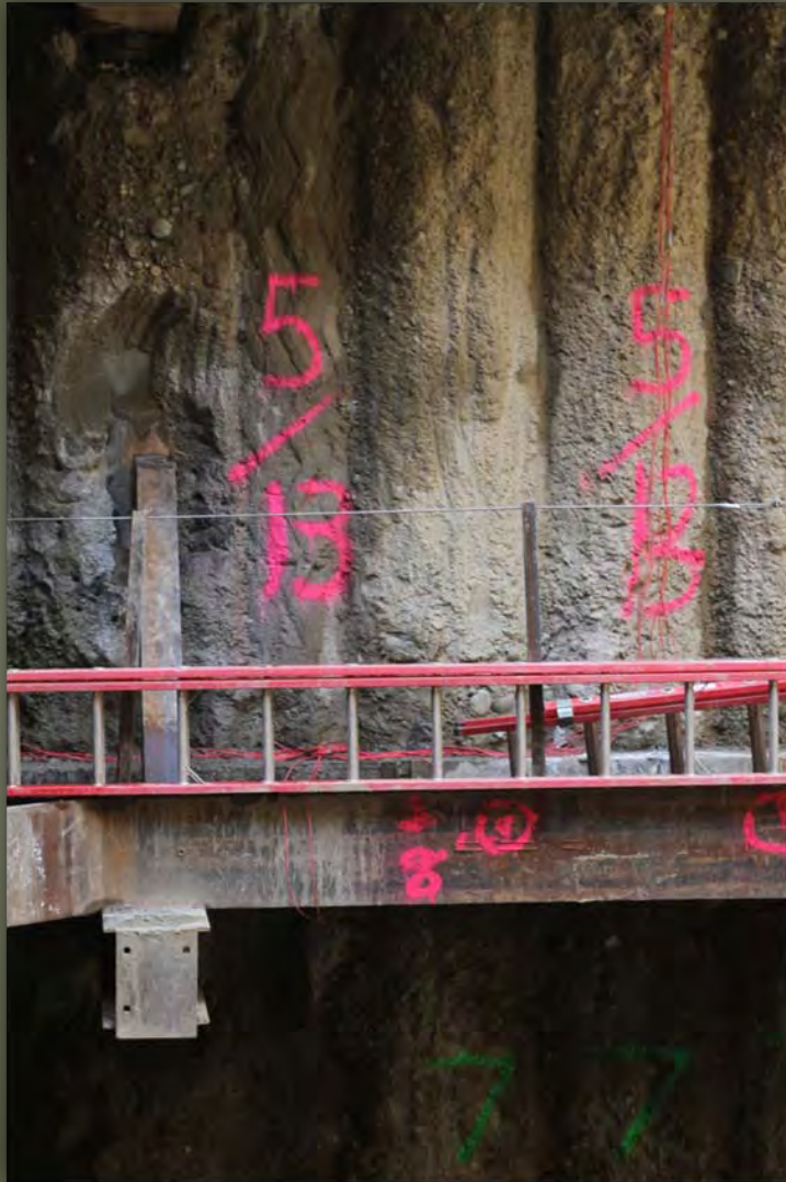
Secant Pile Overlap
