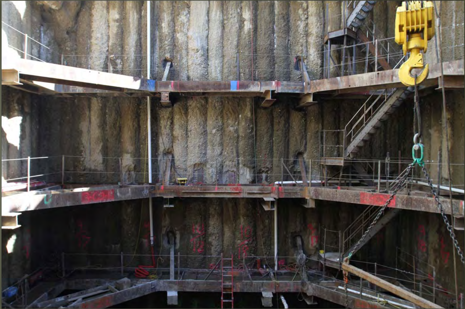
Bracing Levels 2, 3 and 4
