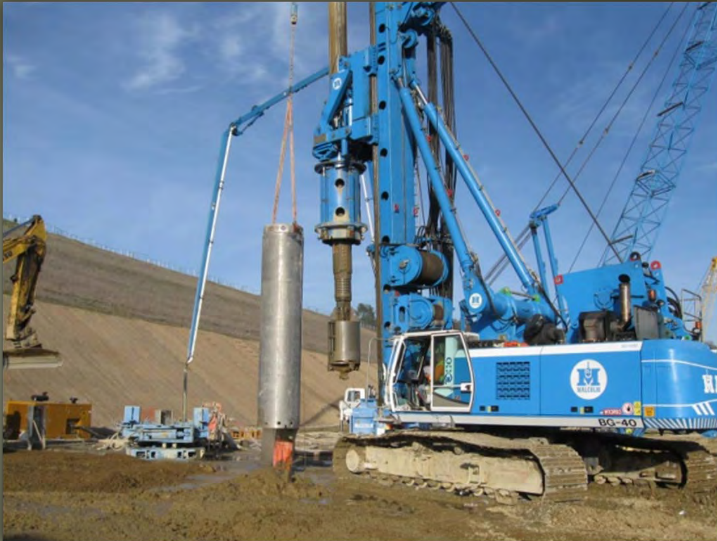
Drill Rig and Casing Oscillator
