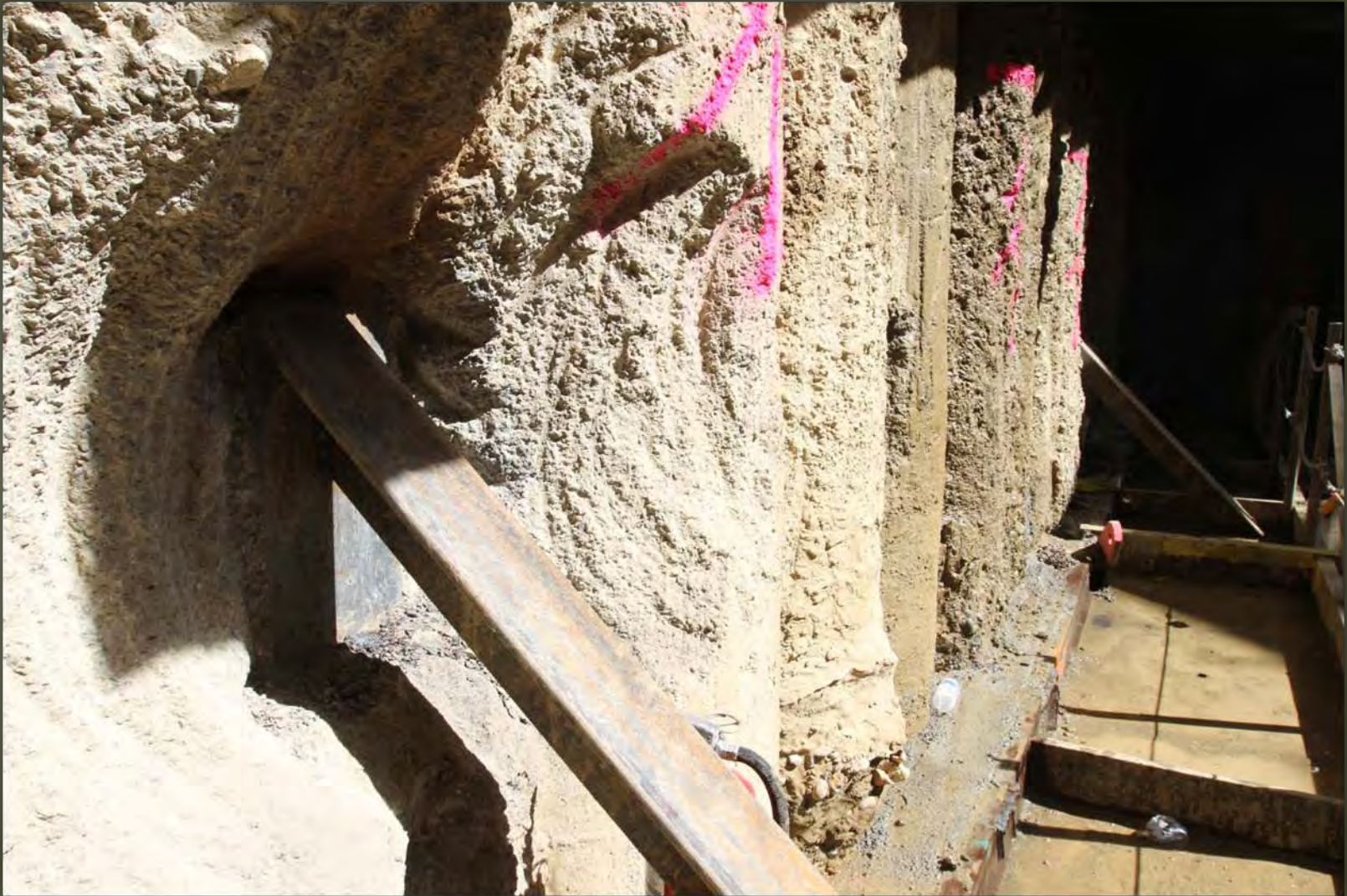
Knee Braces and Concrete Packing
