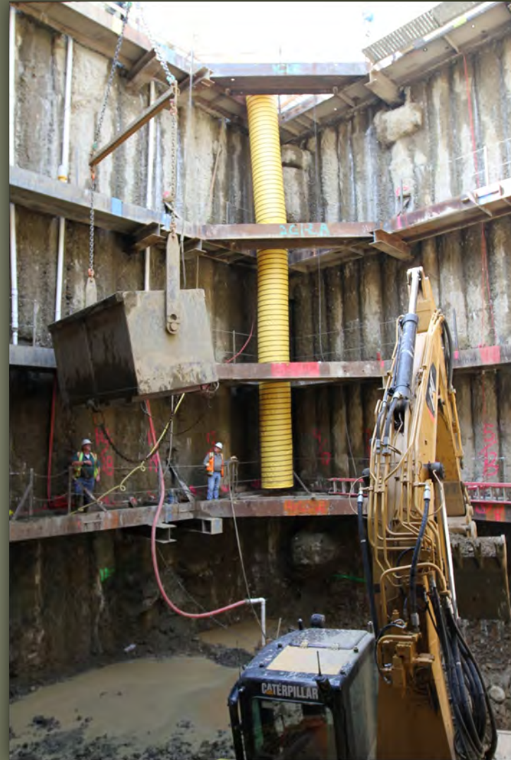
Muck Box Being Used to Remove Soil
