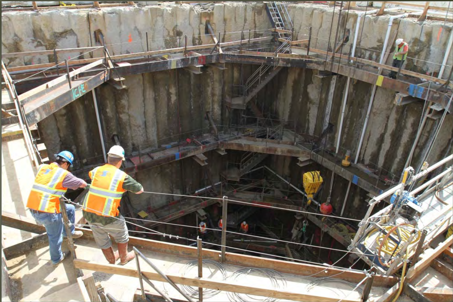
View from Top of Test Section Excavation
