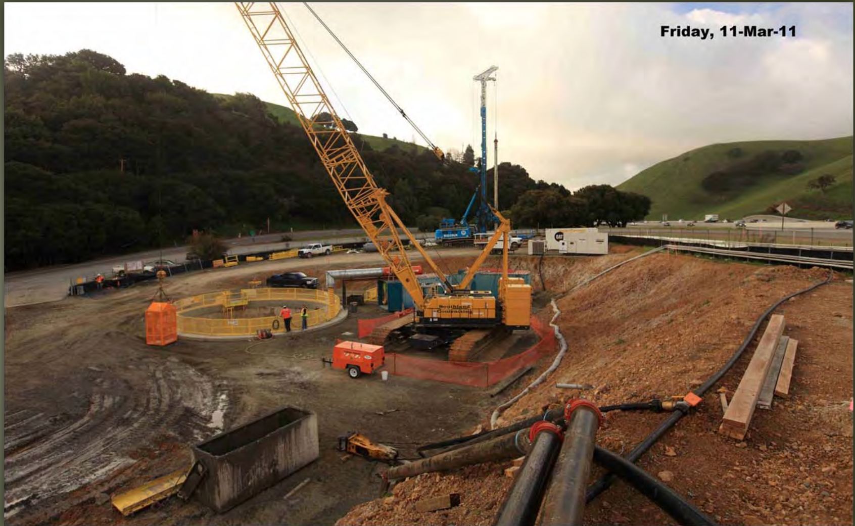
View of Shaft Collar Looking South
