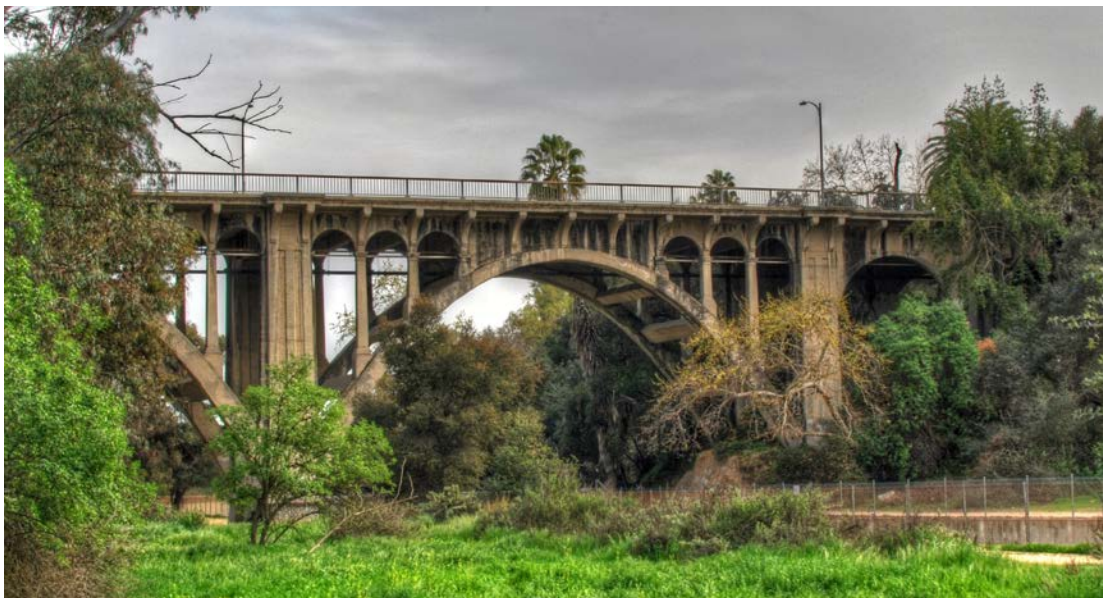
Figure 1 – Original La Loma Bridge
