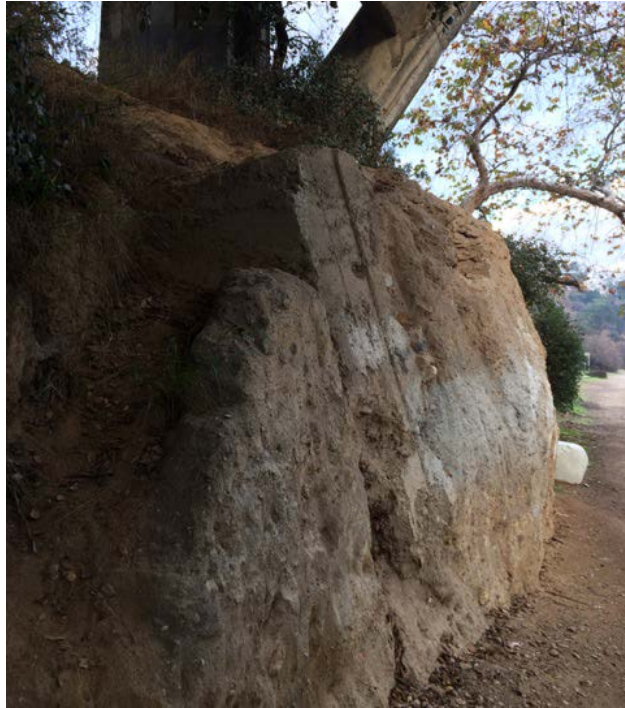
Figure 6 – Pre-construction Conditions at Pier 2 (Topanga Formation)
