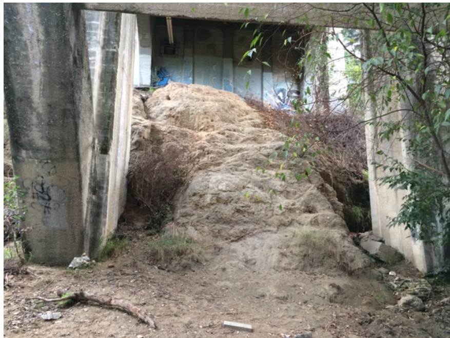
Figure 5 – Pre-construction Conditions at Pier 4 (Quartz Diorite)
