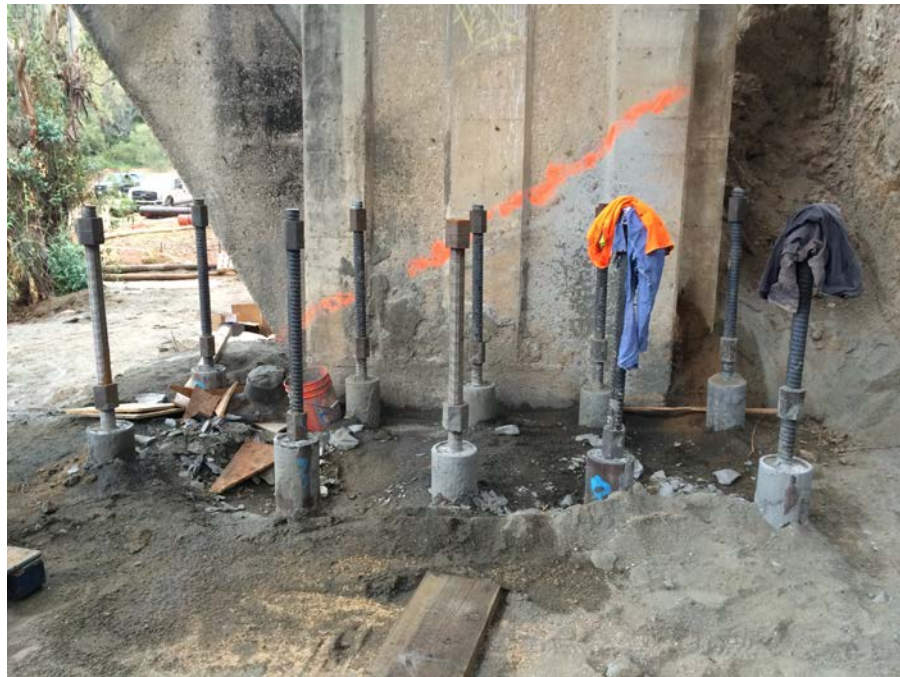
Figure 11 – Completed Micropiles at Pier 2
