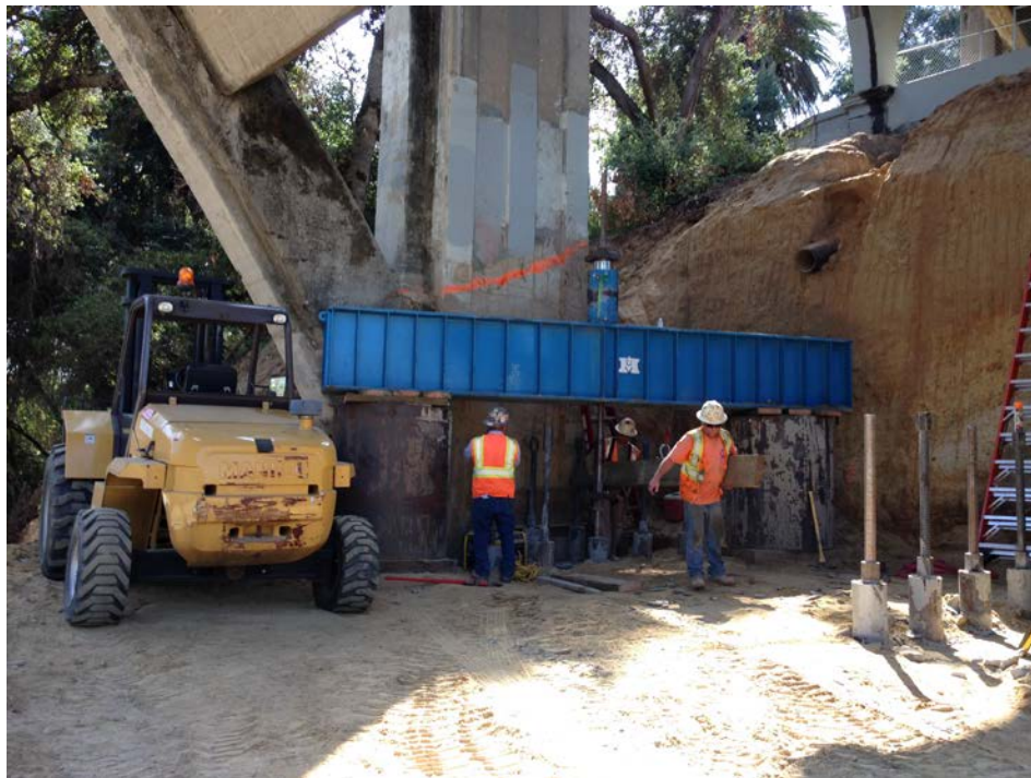
Figure 14 – Proof Test Set-up
