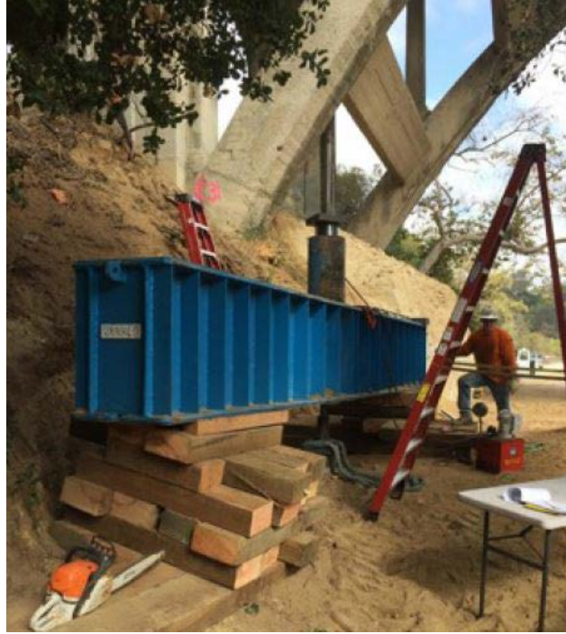
Figure 13 – Pier 2 Verification Test Set-up
