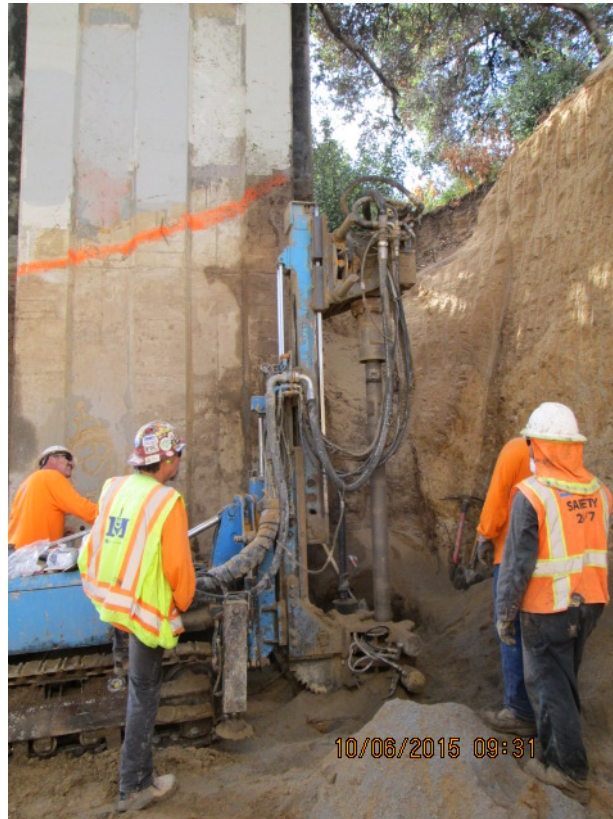
Figure 9 – Micropile Installation
