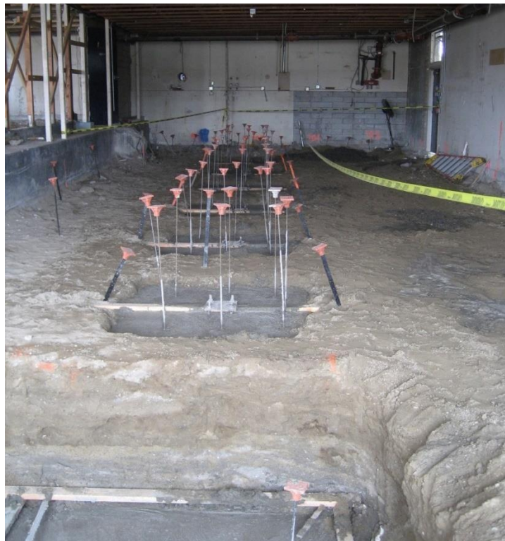
Fig. 5. Spreading footings were cast in the chemical grouted sands.
