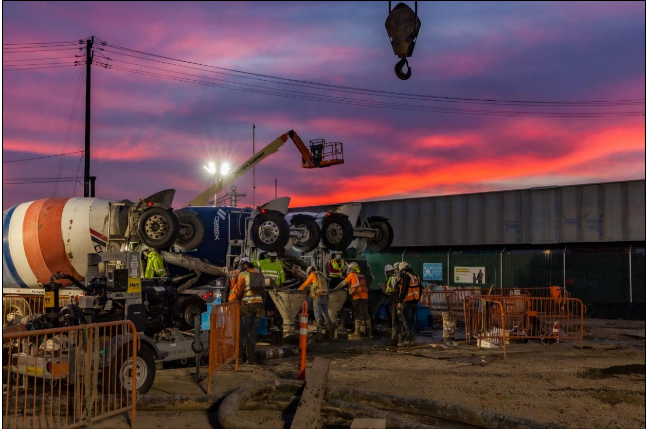
Fig. 16. Primary Panel concrete placement with simultaneous excavation in background.
