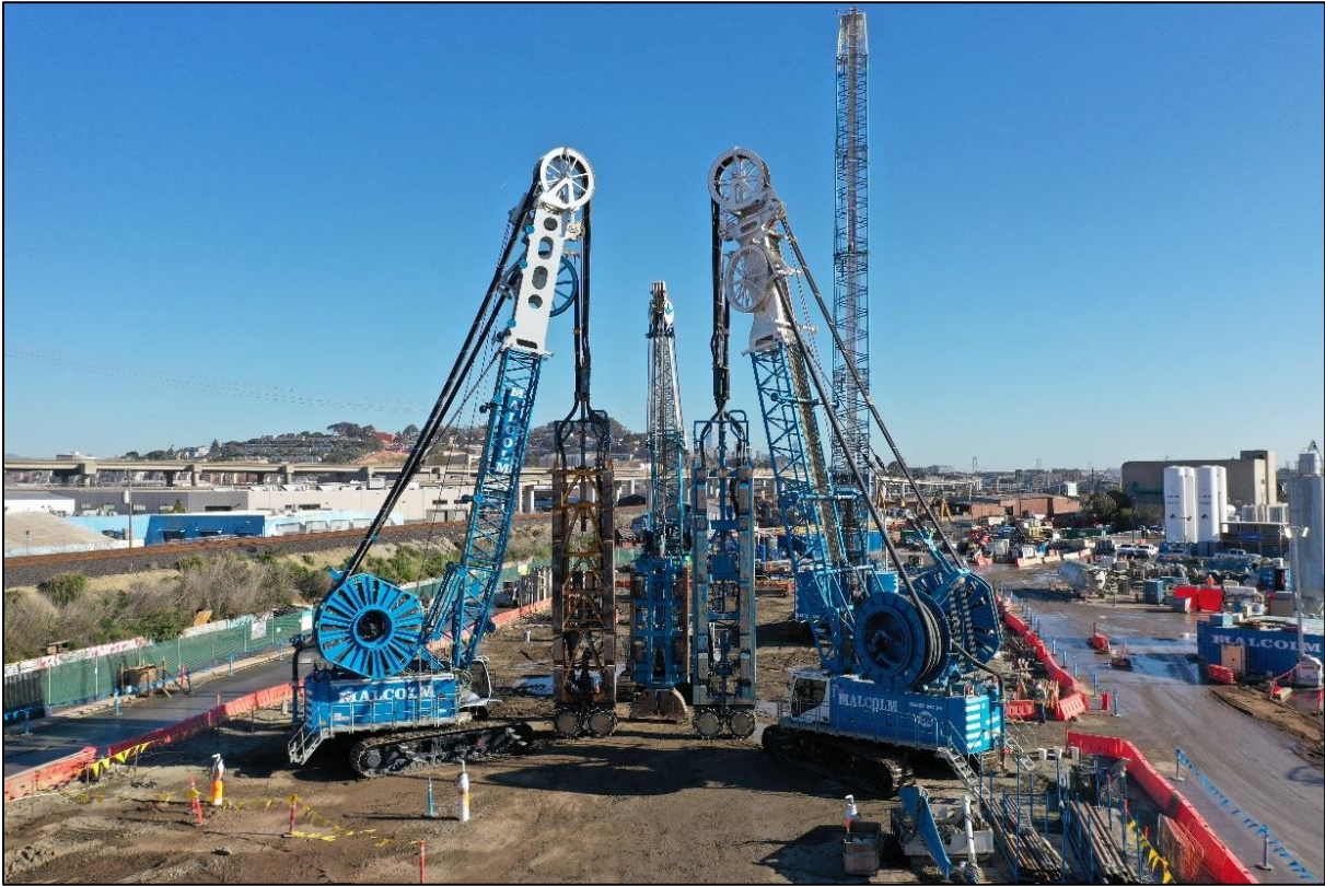
Fig. 13. Two Hydro cutters and One Hydraulic grab
