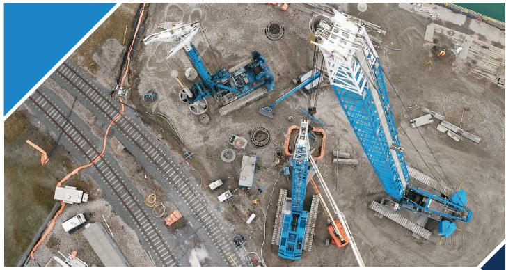
Each main tower pier shaft took approximately 4 to 5 days to complete, and the smaller shafts took about 2/3 as much time. Quality assurance testing took place within about 2 weeks of installation of each shaft. Work took place throughout the winter of 2019, continuing into early 2020. By the beginning of March 2020, only tower pier shafts remained to be built.
