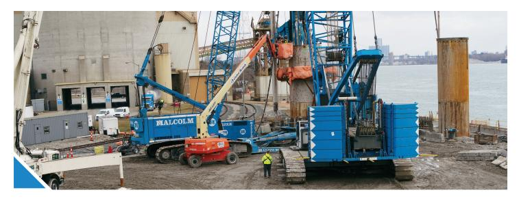
Six back span piers also were designed to be supported by drilled shafts 3 meters in diameter. These piers would be socketed 4.8 meters into rock to resist uplift from the superstructure. The back span piers were located about 1,000 feet to the west of the main bridge piers.
