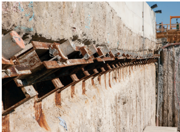
CSM wall with tieback anchors (photo by Mike Butler and Dan Riebe)
