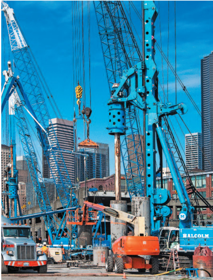
SR99 Tunnel Project, Secant Pile Walls, Seattle, Washington.
