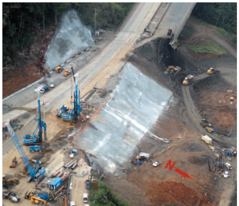
Installation of tangent piles in the Republic of Panama.
