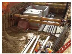
Groundforce hydraulic struts support sheet pile shoring system, providing safety to project teams.
