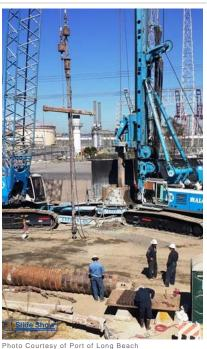
Crews use a novel surface casing removal process to remove old oil wells.
