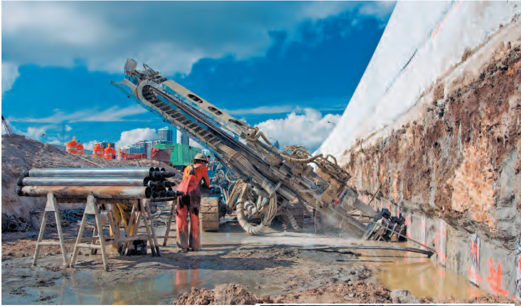
Tieback installation using dual rotary drilling.
