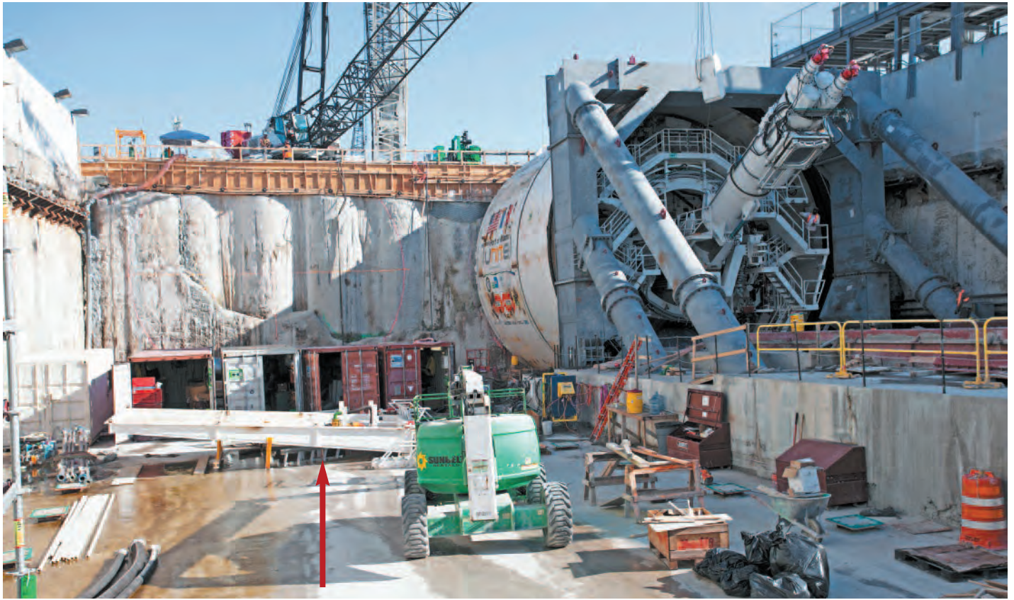
The TBM cutting head assembly.
