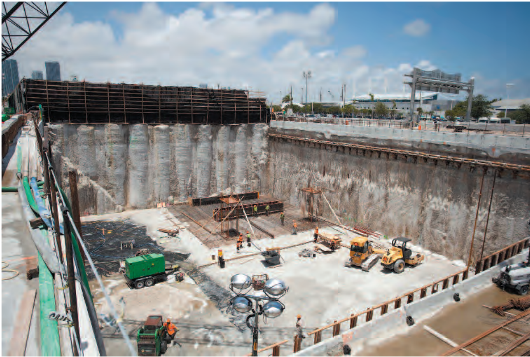
SOE walls made of CSM panels and 12ft secant piles
