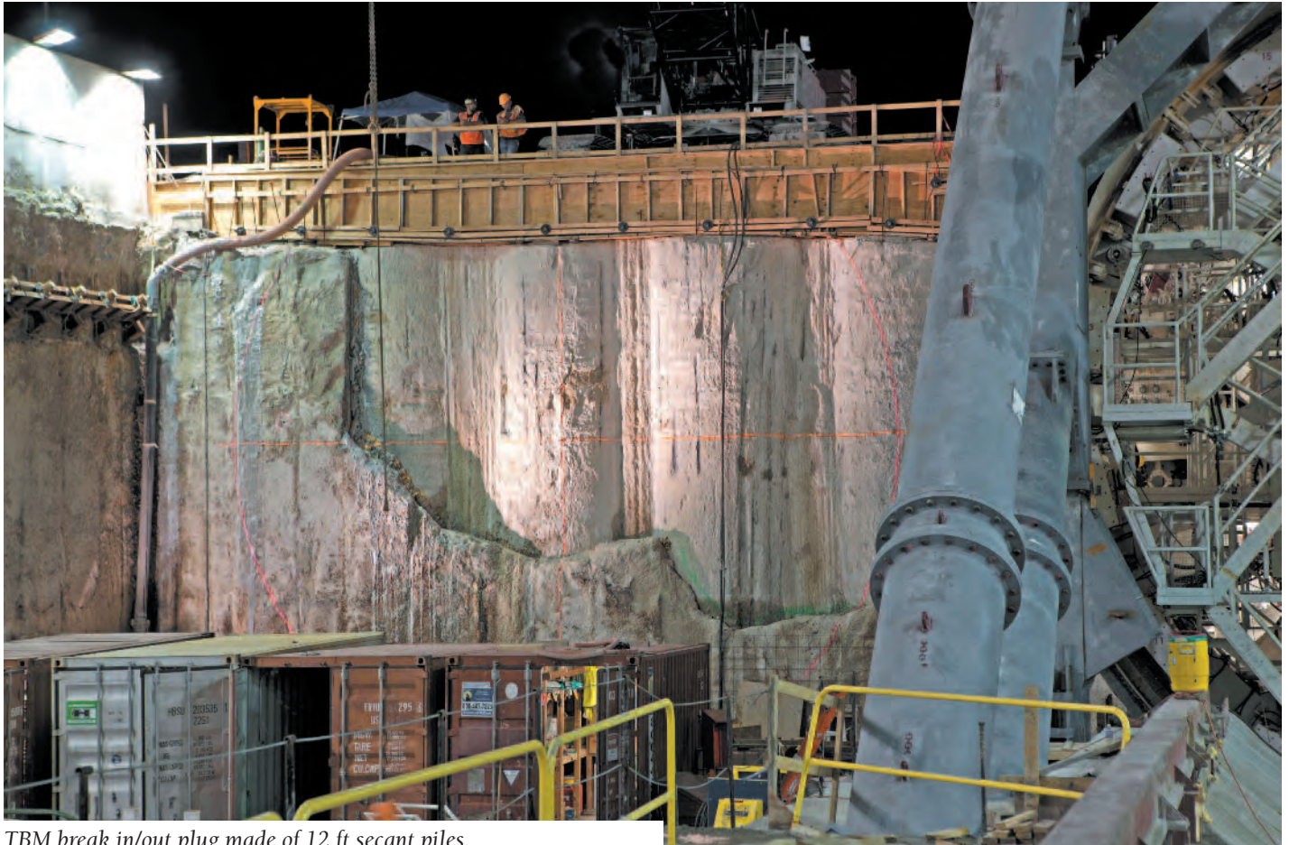
TBM break in/out plug made of 12 ft secant piles.
