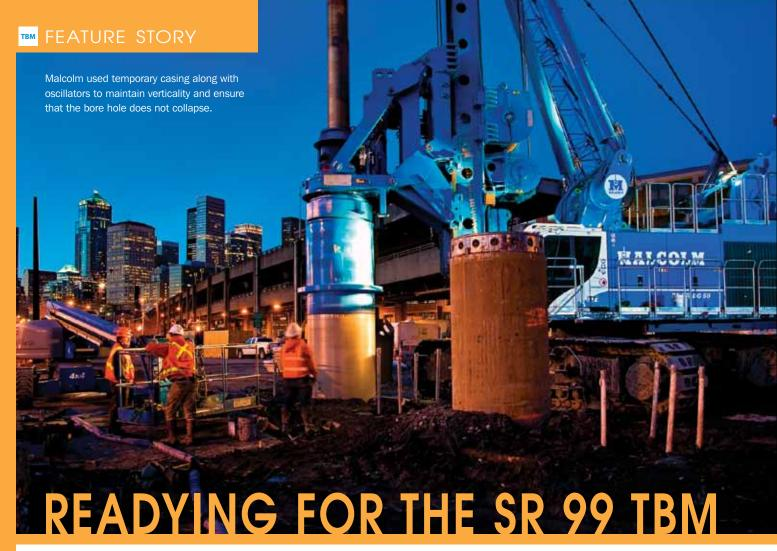
he world's largest TBM gets a lot of the attention when the SR 99 tunnel project in Seattle is discussed. Let's face it, a 57.5-ft diameter machine tends to turn heads. In preparation for the machine's arrival, crews are busy building a massive launch pit south of downtown from which "Bertha" the massive TBM will begin her push.
