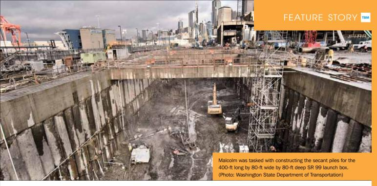
casing should they be encountered. When the piles are drilled to the depth, the casings are extracted during tremie concrete placement ensuring a positive head of concrete is maintained above the bottom of the casing during withdrawal. The fully cased method of pile construction ensures a virtually flaw-free pile, Tucker said.
