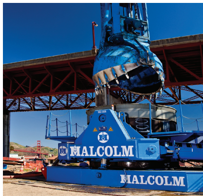
Malcolm Drilling installs large-diameter oscillator shafts in San Francisco.
