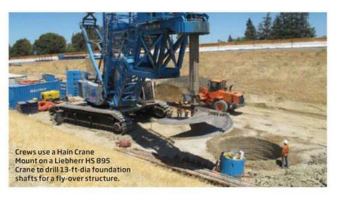
to a depth of 60 ft—an impressive sight for commuters. The location of all three bridge foundations involves working with very dry and loose overburden material and the implementation of a uniquely designed 15-ft-dia support ring to stabilize the 13-ft-dia drilled foundation shafts. In addition, single point soil mixing to a depth of 40 ft was used to stabilize dune sand material and
