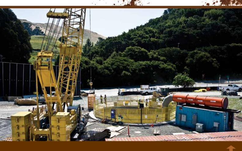
For secant piling, installation tolerance is critical to project success and directly related to cost. When tight tolerances are maintained, pile spacing is maximized, reducing the number of piles required along an excavation perimeter. Once the permissible tolerance is defined, the pile installer must select construction procedures and equipment to satisfy this controlling performance criterion, while minimizing unit construction costs, typically by maximizing production rates.
