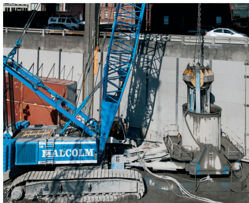
Liebherr HS 895 crane installing large diameter shafts
