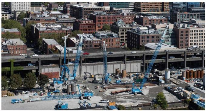
ining on Seattle's SR99 tunnel began in July of 2013. Initial mining progressed slowly through a 4.5 m (14.9-ft) thick fiber-reinforced concrete headwall before immediately entering the first of three planned safe havens. Once through the headwall and safe haven the machine would move through roughly 122 lineal m (400 ft) of jet grout improved soil at a rate of slightly more than 1.6 m/d (5.3 ftpd). It was anticipated
