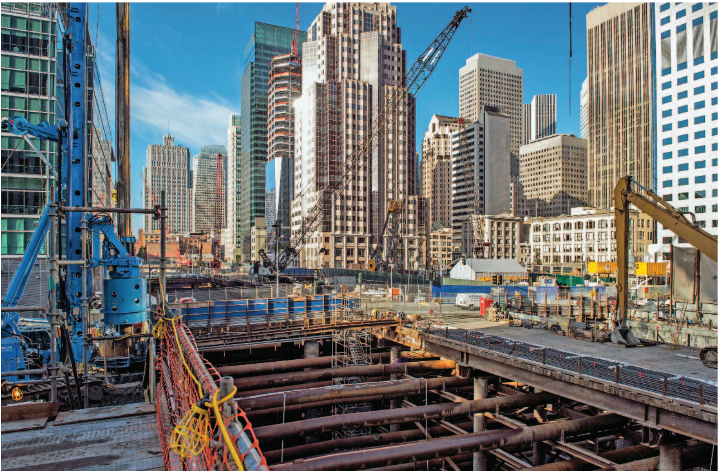
Adjacent Transbay Terminal Project with shared Shoring Wall.
