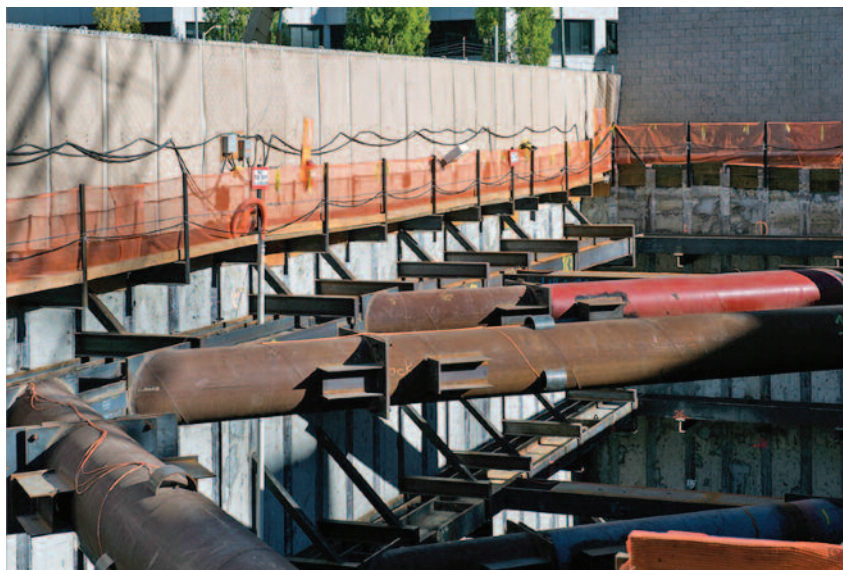
Internal Pipe Struts.
