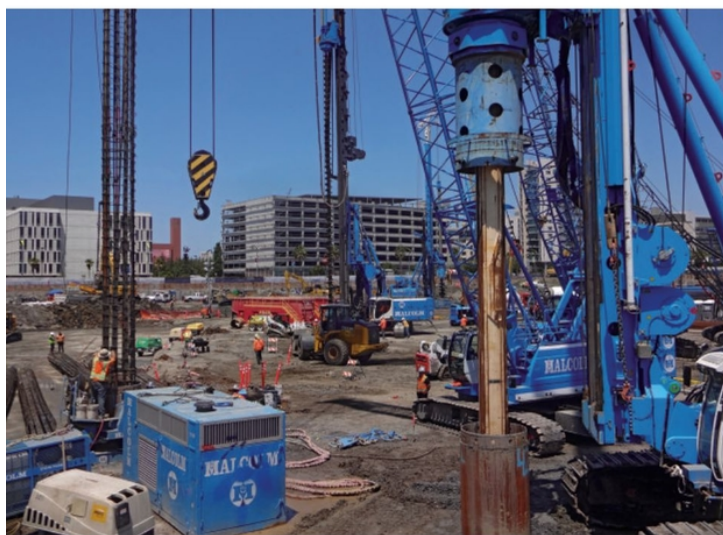
Installing drilled shafts and ACIP piles
