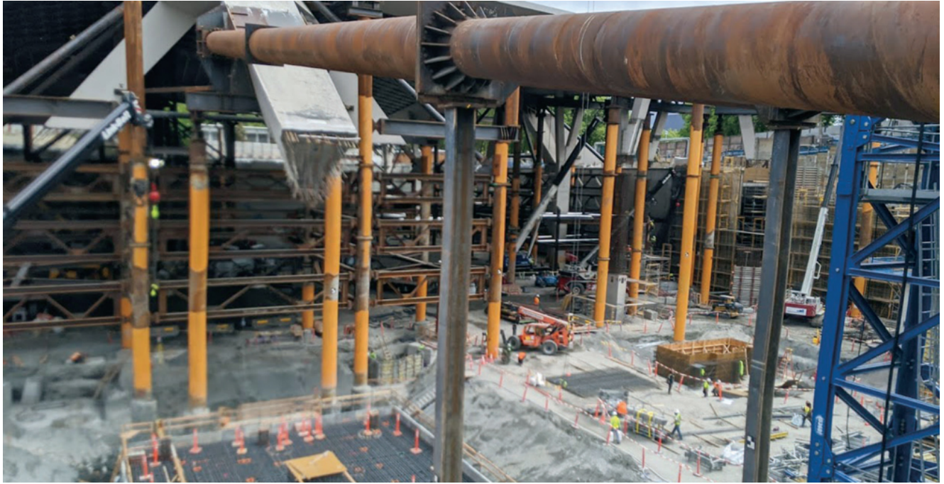
MALCOLM/DBM INSTALLED A TANGENT WALL TO FACILITATE ROOF LATERAL LOAD TRANSFER
