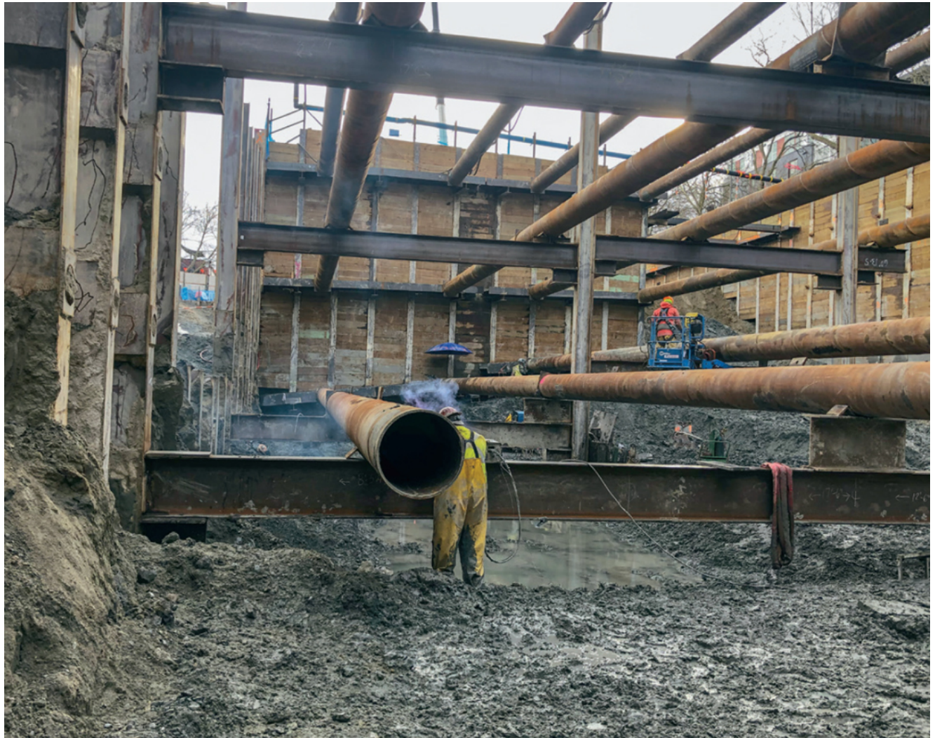
A MALCOLM/DBM PILEBUCK WELDS THE WEST TEMP RAMP BRACING ELEMENTS ON SITE
