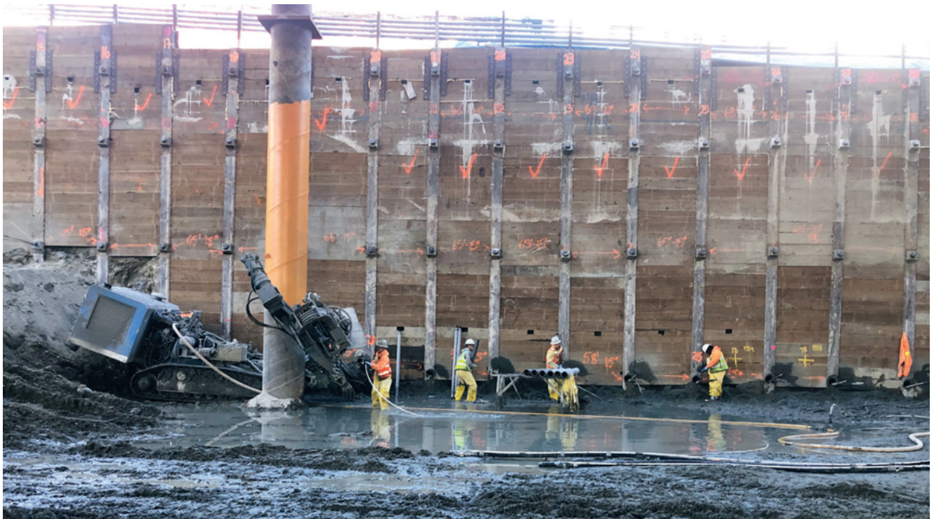
MALCOLM/DBM EQUIPMENT CONFIGURED TO INSTALL TIEBACK ANCHORS AROUND TEMPORARY ROOF SUPPORT COLUMNS
