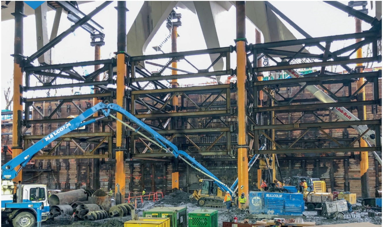
INSTALLING SHAFTS AROUND THE PREVIOUSLY INSTALLED TEMPORARY ROOF SYSTEM BRACING
