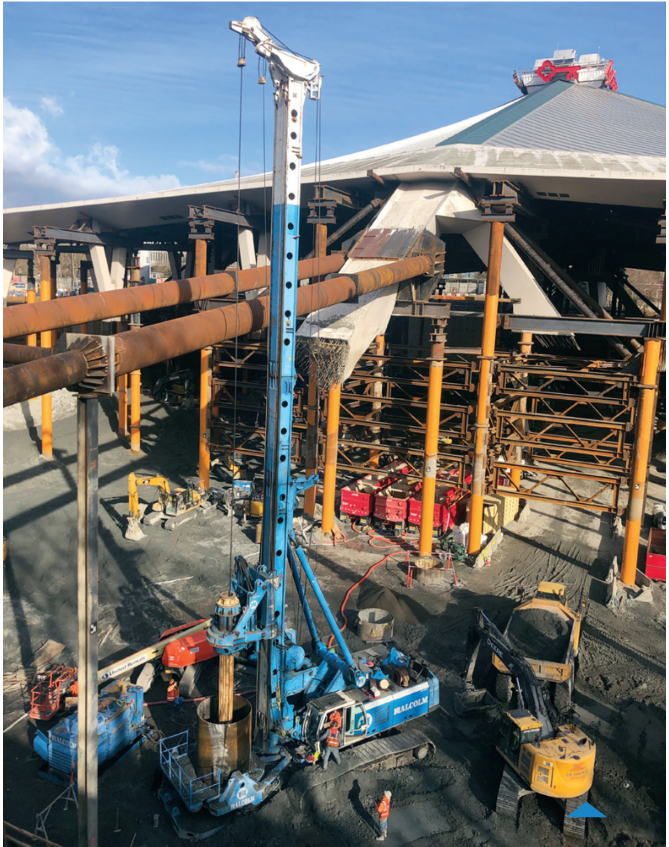
PERMANENT FOUNDATION SHAFTS BEING INSTALLED ADJACENT TO AND UNDERNEATH TEMPORARY ROOF SUPPORT BRACING
