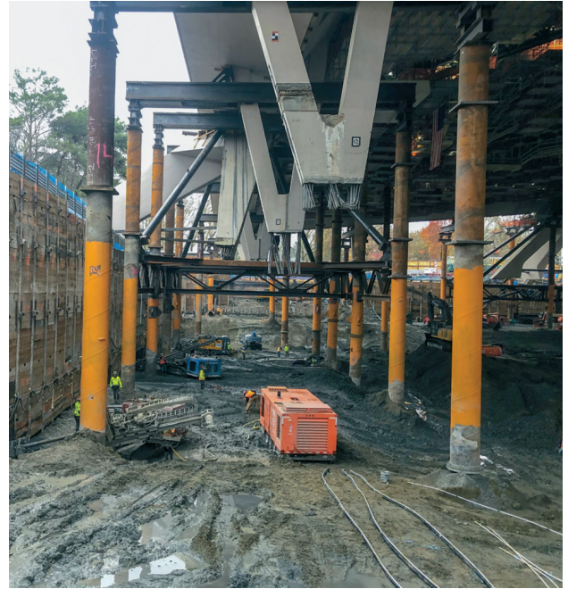
ONCE THE TEMPORARY ROOF SUPPORT SYSTEM WAS INSTALLED, THE ORIGINAL ROOF SUPPORT COLUMNS WERE SEPARATED FROM THEIR FOOTINGS
