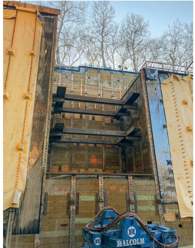
INTERNALLY BRACED SE SNORKEL INCORPORATED INTO PERIMETER SHORING SYSTEM
