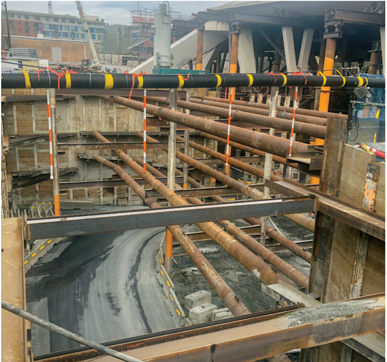
THE WEST TEMP RAMP ALLOWED CONTINUOUS ACCESS INTO THE BOWL WHILE THE MINED TUNNEL WAS BEING COMPLETED
