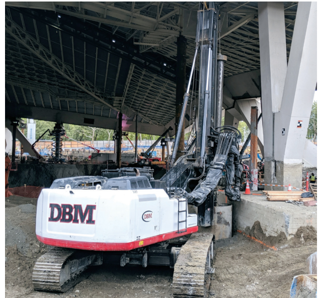
PROXIMITY TO EXISTING ROOF SUPPORT ELEMENTS WAS A CONSTANT CHALLENGE DURING TEMPORARY ROOF SUPPORT SHAFT INSTALLATION
