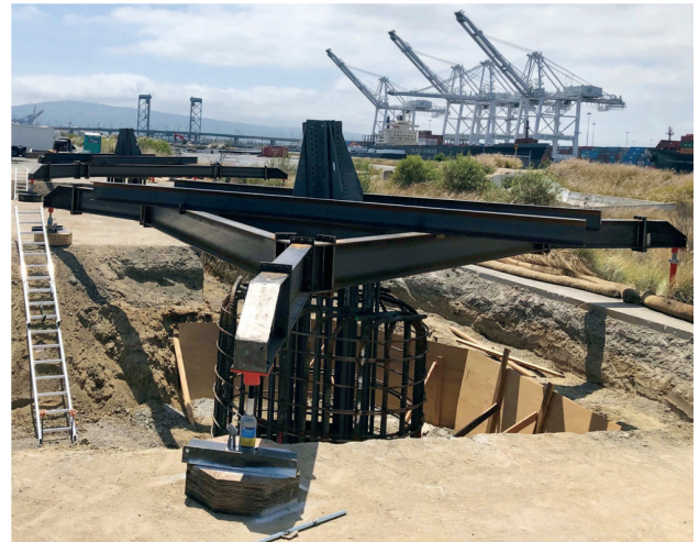
STUB ANGLE AND HEAVY SUPPORTS
