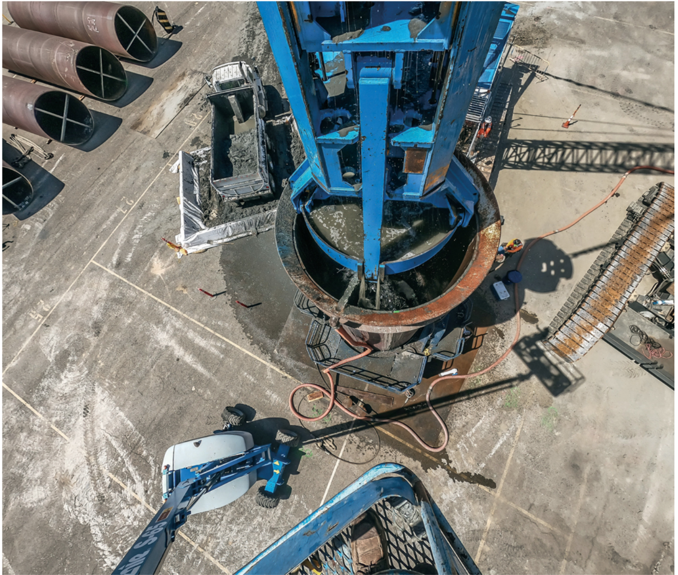
SPHERICAL GRAB EXCAVATION
