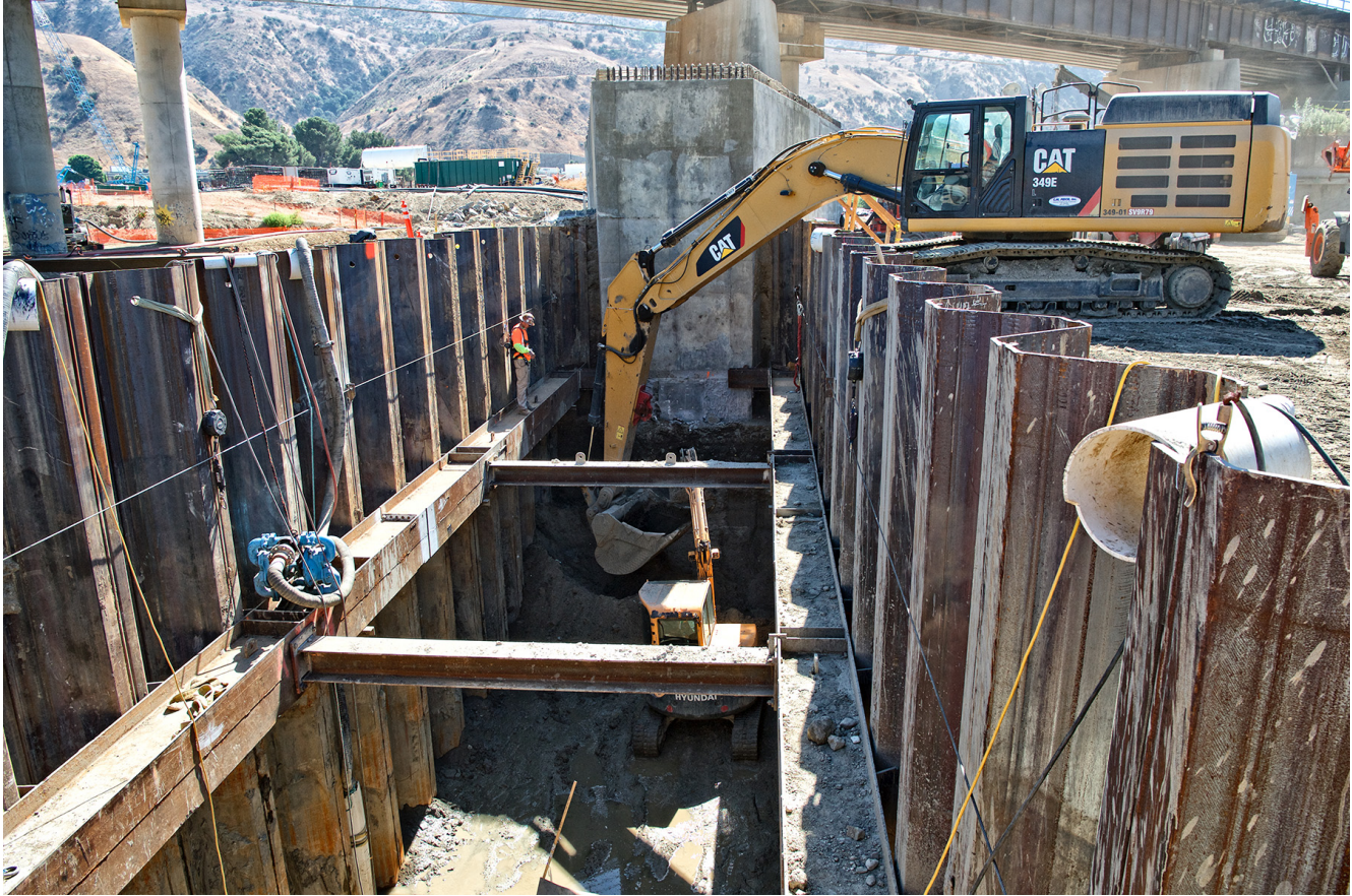
Excavation inside the cofferdams entailed the use of dewatering wells and localized unwatering due to the adjacent river and the highly permeable sandy soils at the site. (Photograph courtesy of Malcolm International LLC)
