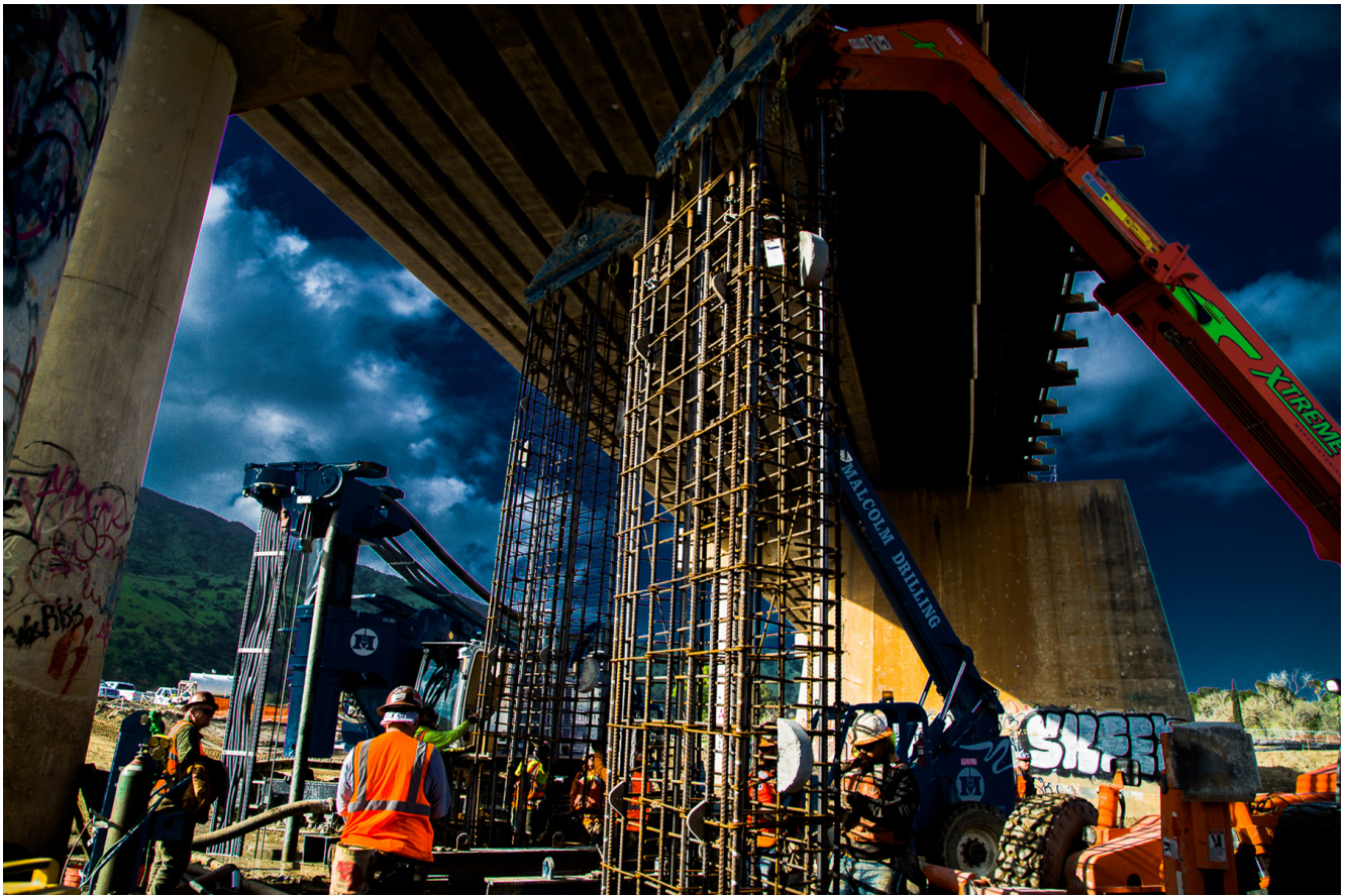
Before the diaphragm wall panels could be installed, panel verticality testing, rebar inspection, and bentonite testing were conducted. (Photograph courtesy of Malcolm International LLC)
