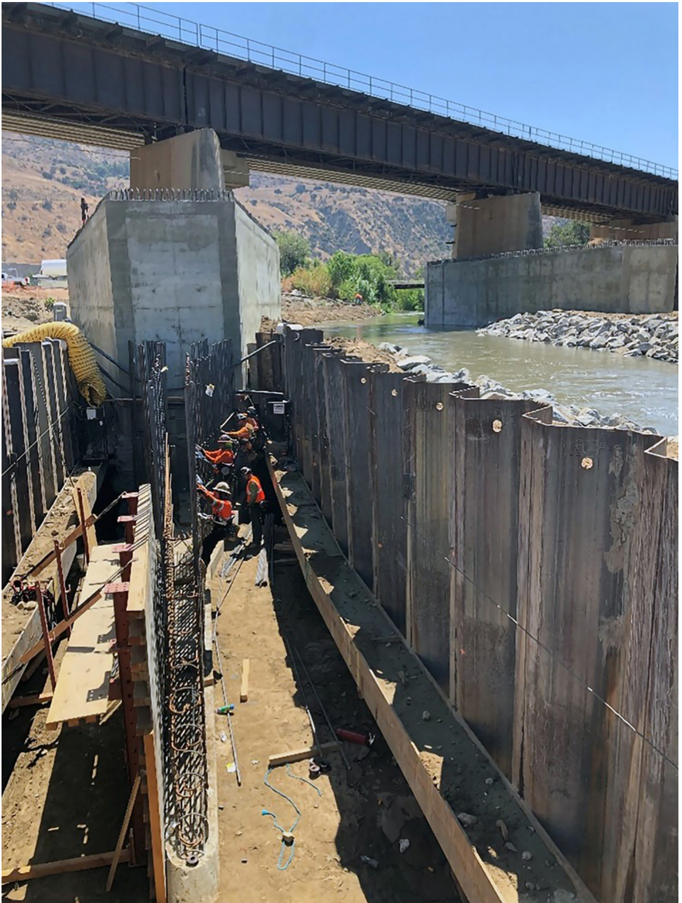
The pier noses, installed inside braced sheet pile cofferdams, feature a tapered shape with rounded edges to allow water to easily pass between pier groups. (Photograph courtesy of Malcolm International LLC)
