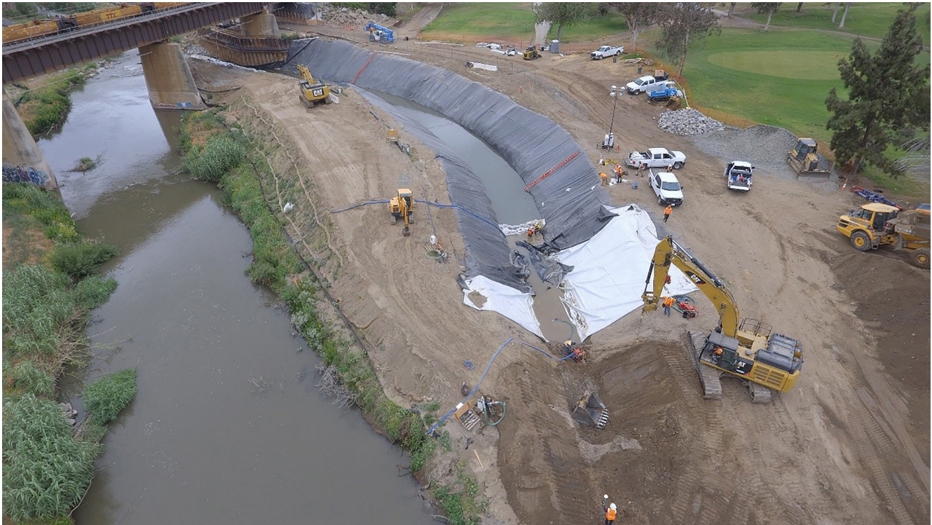
A crew diverted a portion of the Santa Ana River temporarily to accommodate construction of the pier-protection features beneath the bridge. The natural river alignment is on the left. (Photograph courtesy of Malcolm International LLC)
