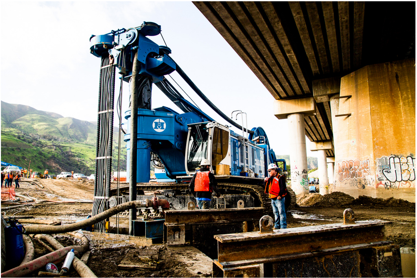
A low-overhead hydro cutter, used to excavate the ground to make room for the diaphragm wall panels, operated within tight tolerances beneath the bridge. (Photograph courtesy of Malcolm International LLC)
