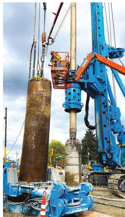
When a tunnel boring machine got stuck at the I-75 modernization project in Detroit, a vertical rescue shaft was created to get the machine named "Eliza" out.
