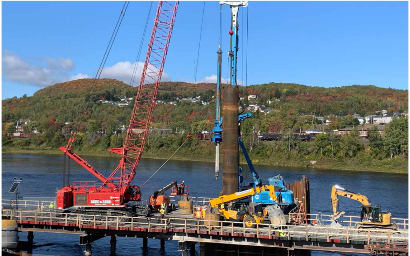
REED & REED ASSISTING MALCOLM DRILLING BY LIFTING AND SETTING THE PERMANENT CASING SECTION FOR MALCOLM'S BG40 TO INSTALL. (PHOTO COURTESY OF AROOSTOOK UNMANNED AERIAL PHOTOGRAPHY)
