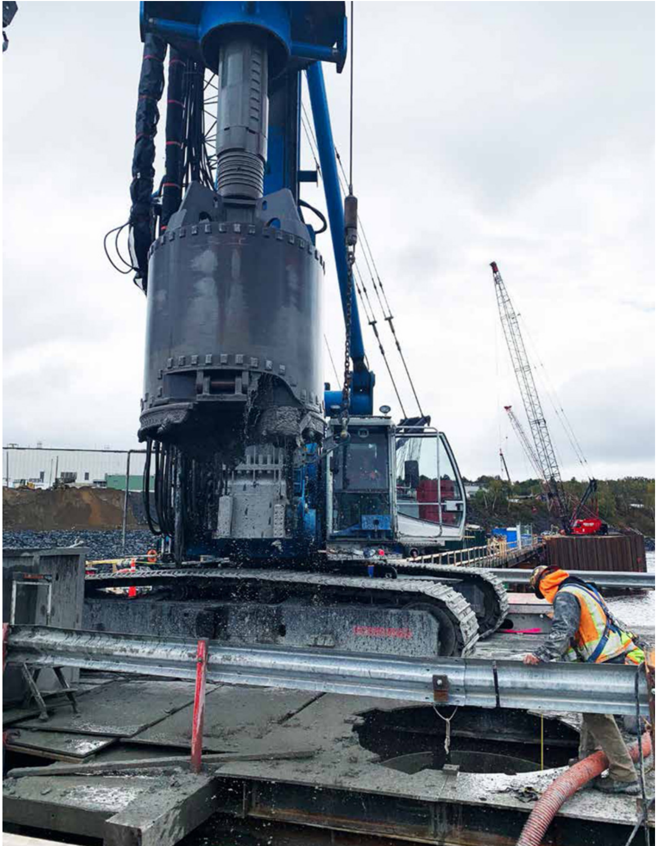
DRILLING SLATE ON THE TRESTLE WORK PLATFORM.
