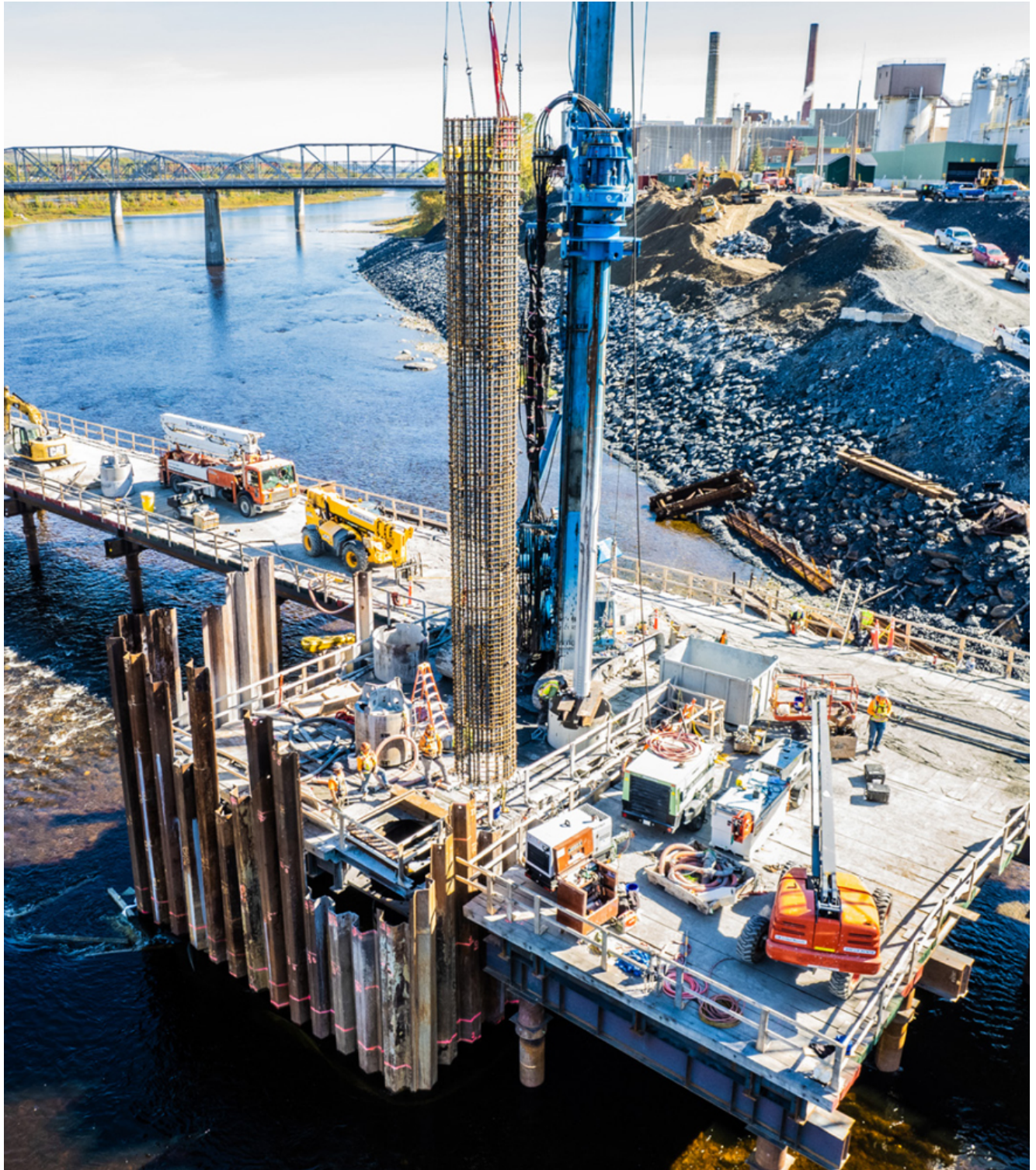
INSTALLING THE REBAR CAGE PRIOR TO CONCRETE PLACEMENT. (PHOTO COURTESY OF AROOSTOOK UNMANNED AERIAL PHOTOGRAPHY)
