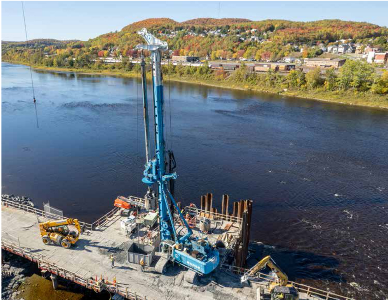
DRILLING OVERBURDEN ON THE TRESTLE WORK PLATFORM. (PHOTO COURTESY OF AROOSTOOK UNMANNED AERIAL PHOTOGRAPHY)
