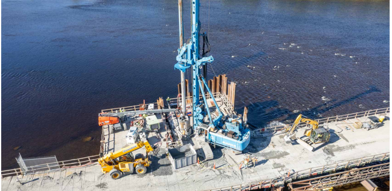
MALCOLM DRILLING INSTALLING DRILLED SHAFTS VIA WORK TRESTLE ON THE ST. JOHN RIVER IN MADAWAKSA, MAINE.
