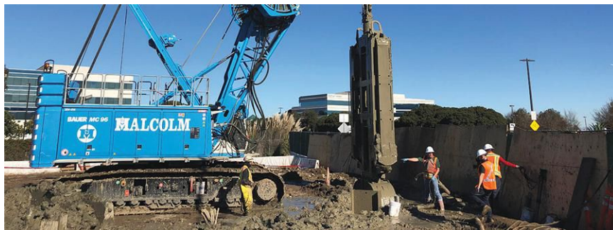
Malcolm is installing slurry wall panels for the Airport Access Shaft.
