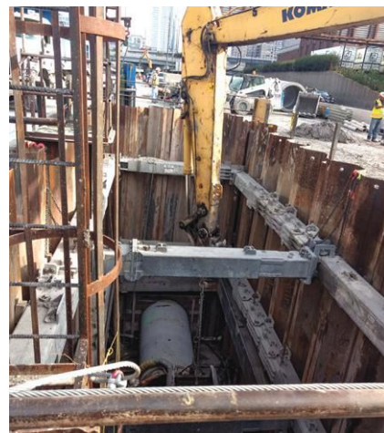
National Trench Safety provides a contractor with a hydraulic bracing system.
