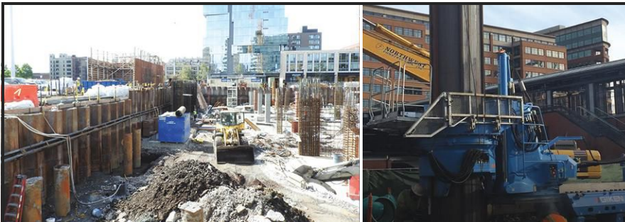
Malcolm Drilling crews utilize a cutter soil mixing (CSM) technique for temporary shoring activities.
