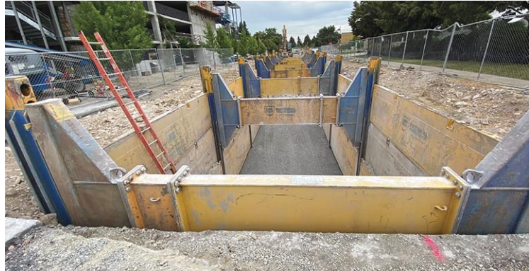
Slide rail shoring systems require no interior wales or beams, which opens up more space for crews to perform excavation and other activities in a trench safely and efficiently.
