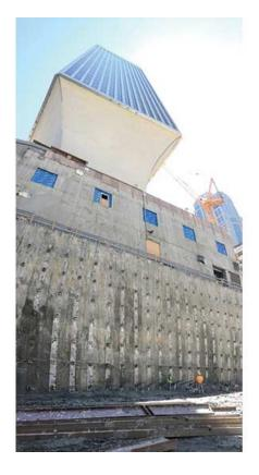
Matyasovszky led the tricky shoring-and-drilling operation that kept a deep pit from undermining a 40-story tower.
